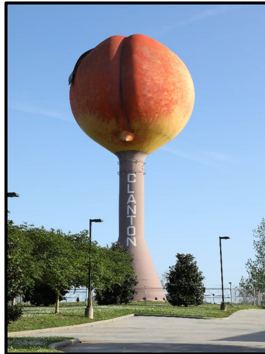
Figure 2. Clanton, Alabama water tower.
