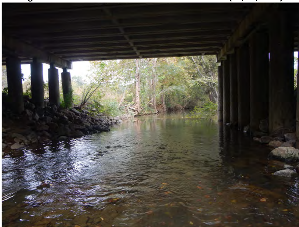
Figure 7.5.2: At Station SHRT-1: Downstream View (10/12/2022)
