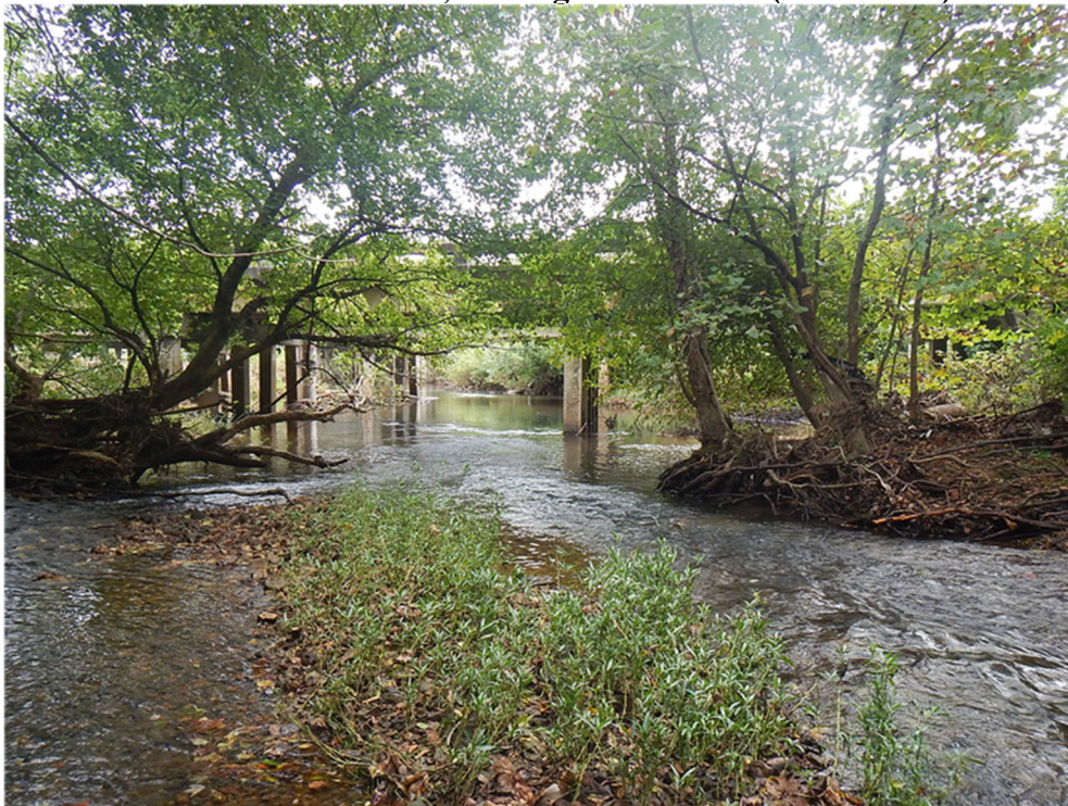
At station INDM-249, looking downstream (10/05/2021)
