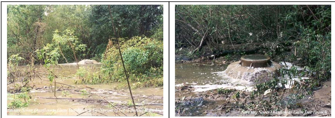
Figure 3-6 Gum Tree Branch Sanitary Sewer Overflows
