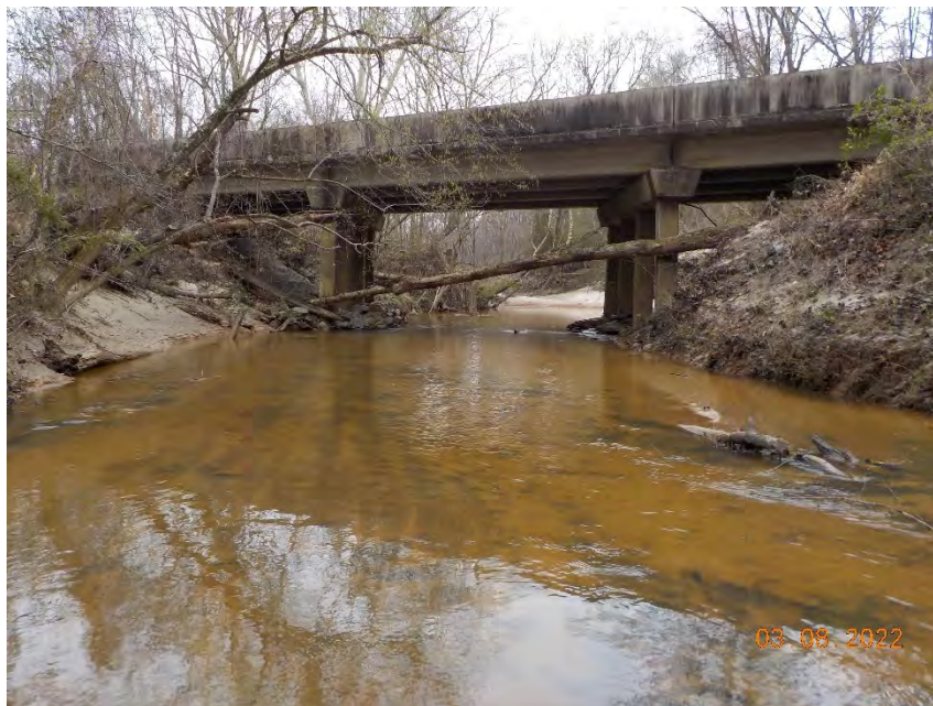
Figure 6. At Station CLEC-1: Downstream View of Clear Creek (3/8/2022)
