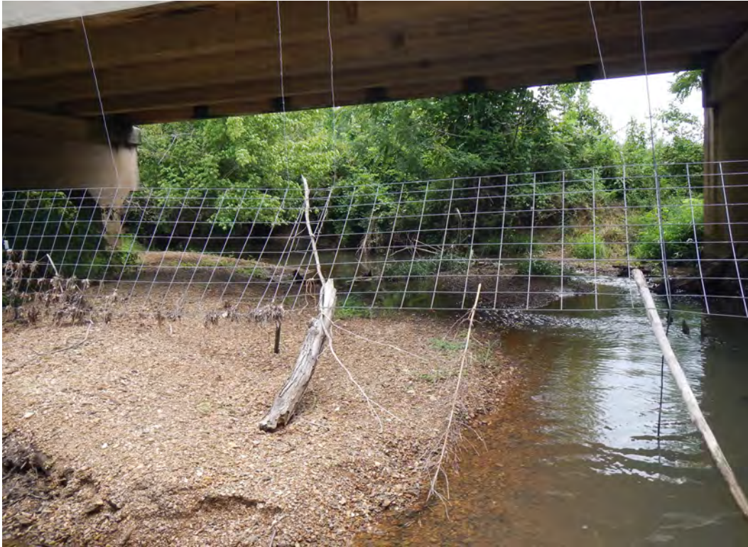
Figure 7.3.3: At Station CHLC-1: Upstream View (8/11/2016)
