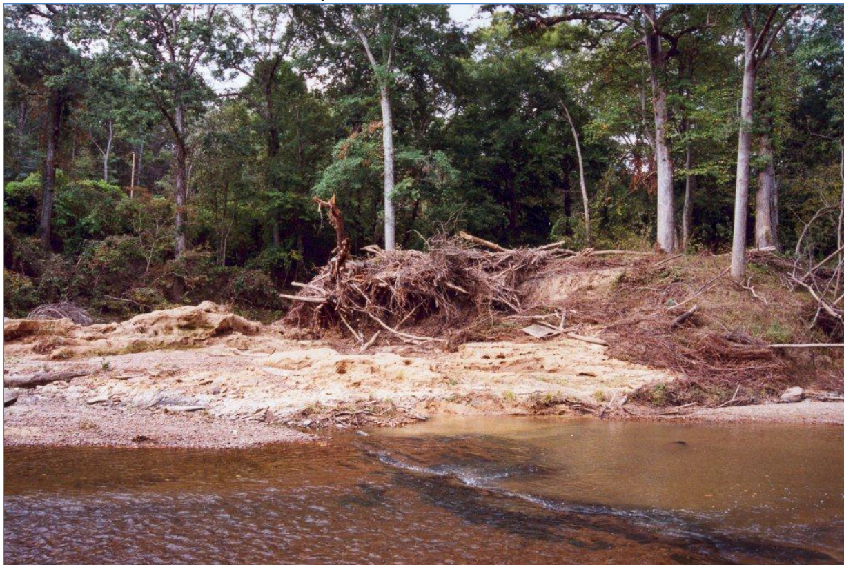
Picture 3-3: Example of an Unstable Bank on the Cahaba River
