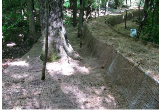
Figure SB-1 Sediment Retention Barrier
