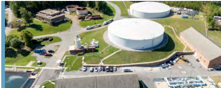
Pictured: Award-Winning Shades Mountain Filtration Plant
