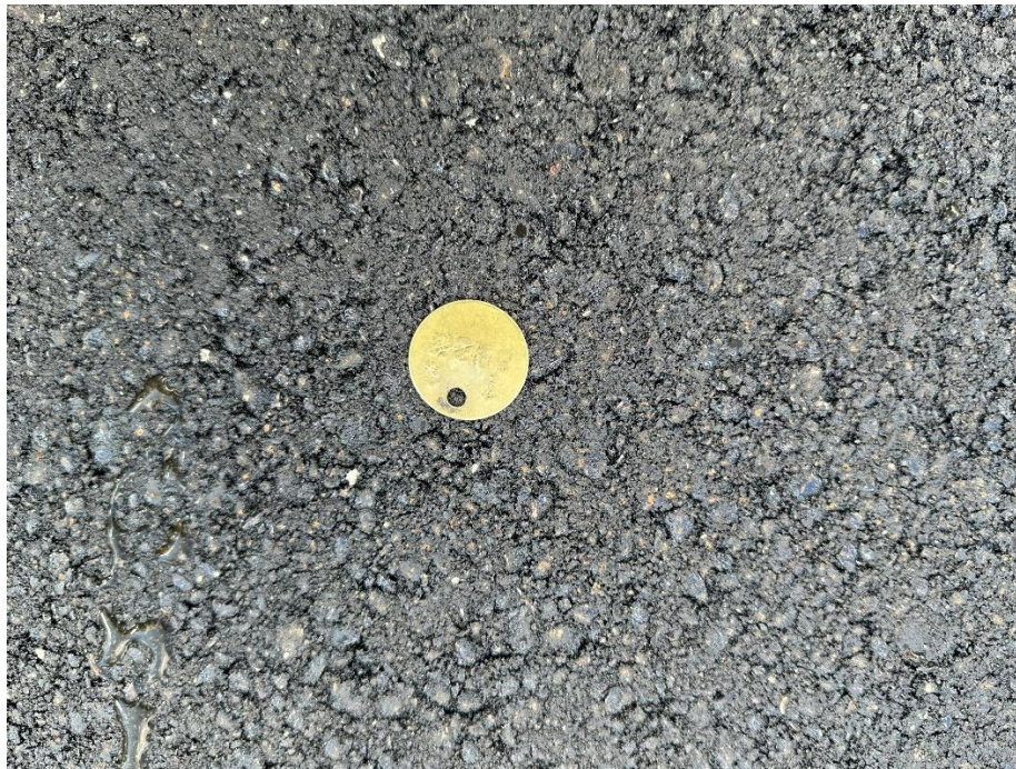
Figure 5. Close-up of GTR Section after Placement and Compaction
