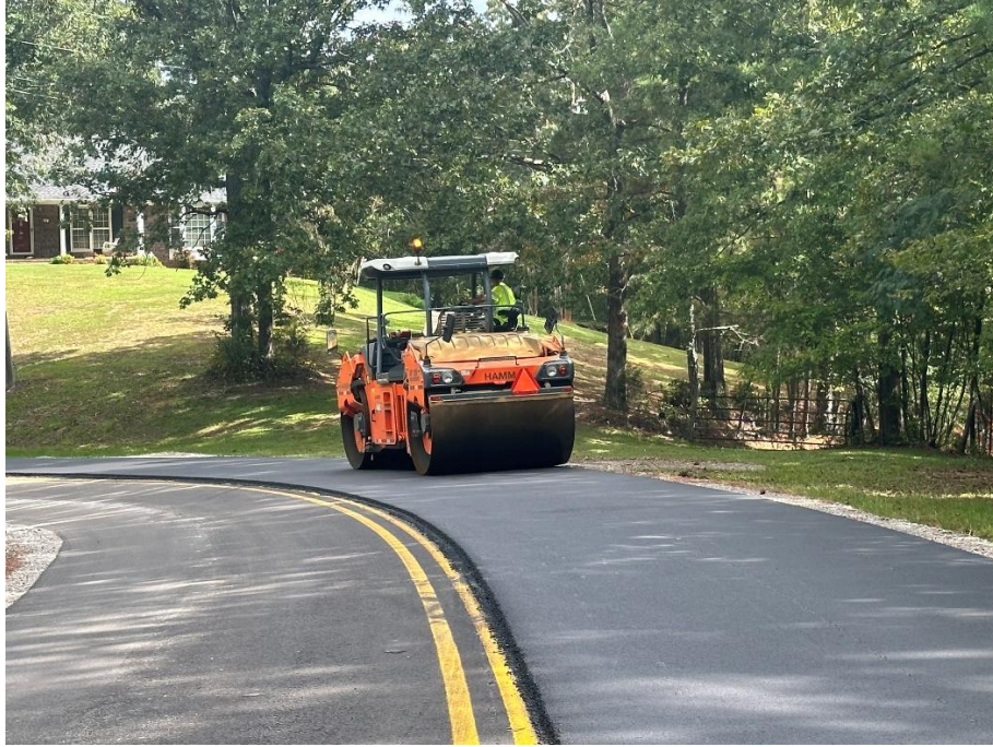
Figure 4. GTR Mix Compaction
