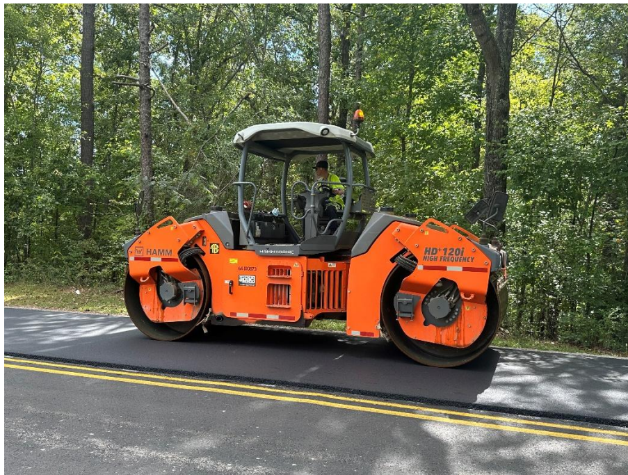
Figure 3. GTR Mix Compaction
