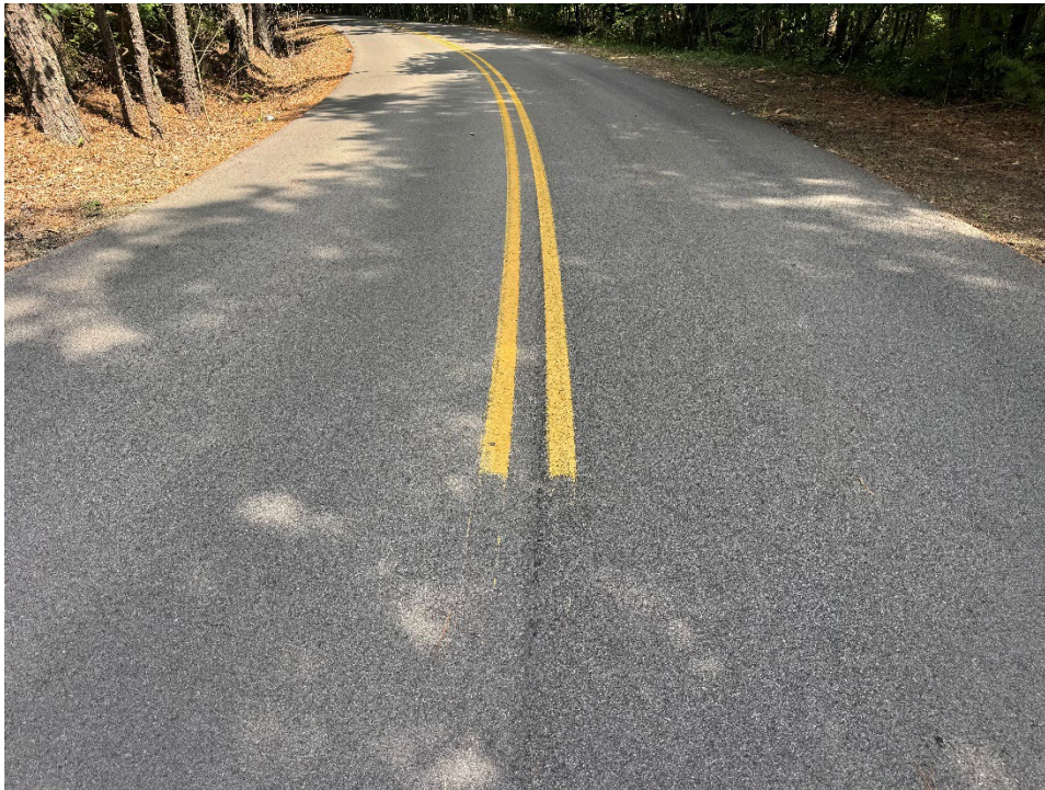
Figure 2 Example of Both Mixes at Two-Year Inspection (Rubber on Left, Control on Right)
