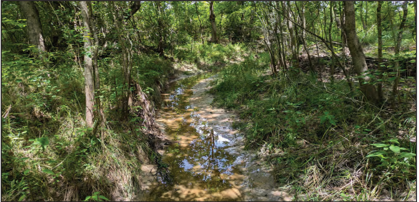
Looking upstream toward the end of Ditch 1.
