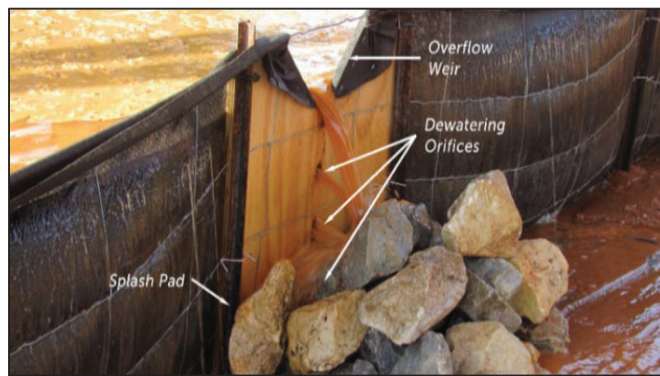
Figure SB-2 Example dewatering board & overflow weir.
