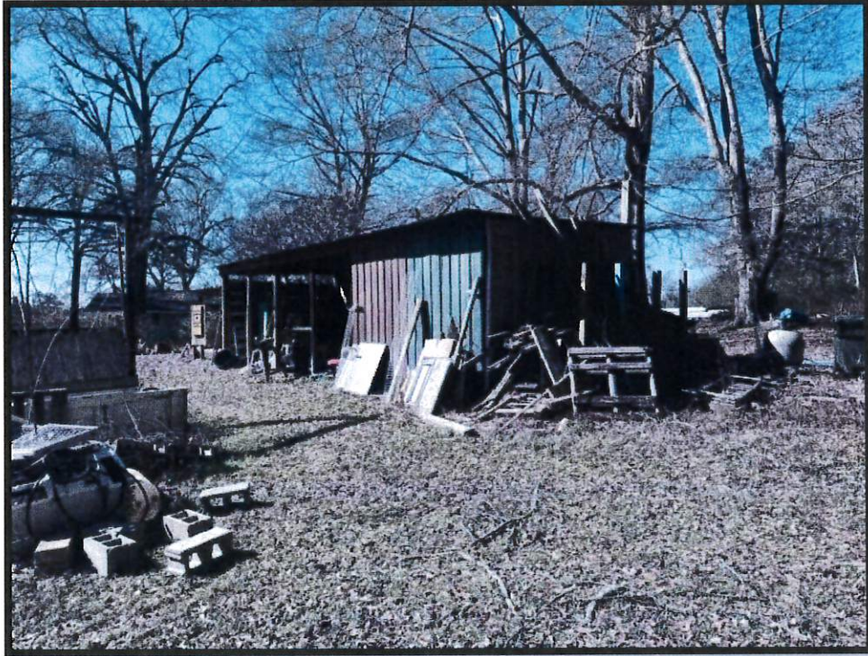
Photograph 11: Storage/Maintenance shed located centrally on Subject Property.
