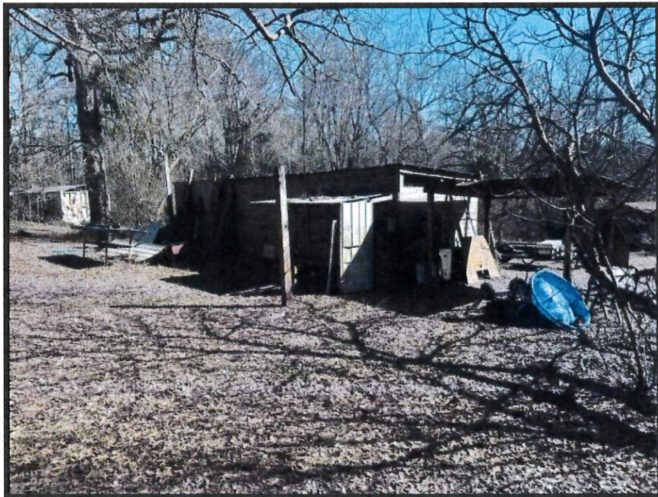
Photograph 12: Storage/Maintenance Shed located centrally in Subject Property.
