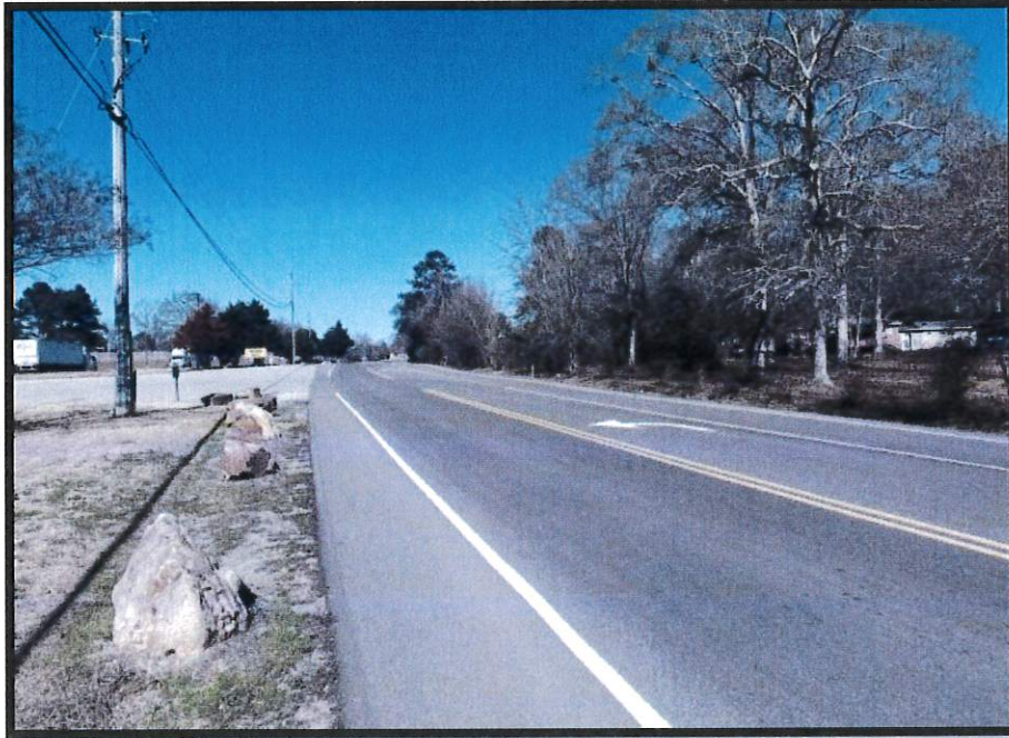
Photograph 3: View of CR-764 with western border of Subject Property on right side of road.
