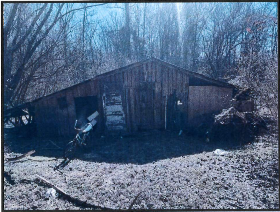
Photograph 19: View of derelict barn located centrally on Subject Property.
