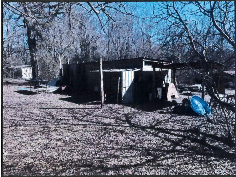
Photograph 12: Storage/Maintenance Shed located centrally in Subject Property.
