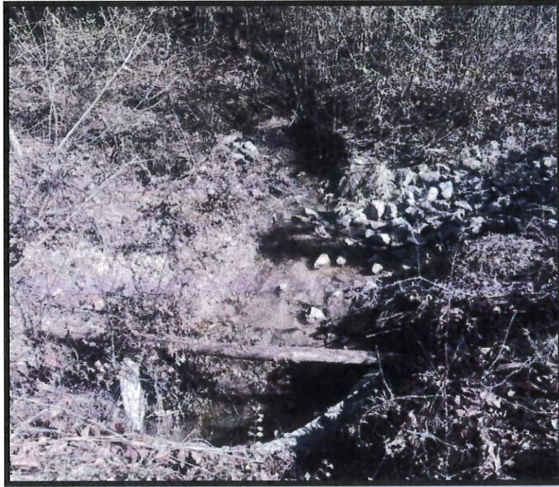
Photograph 15: Creek outlet on SW corner of Subject Property.
