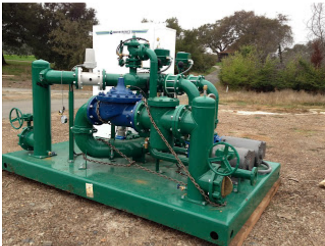
New golf course pump station ready for install!
