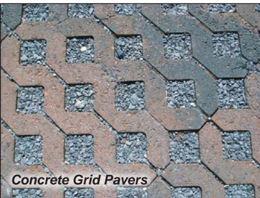
Permeable Interlocking Concrete Pavers
