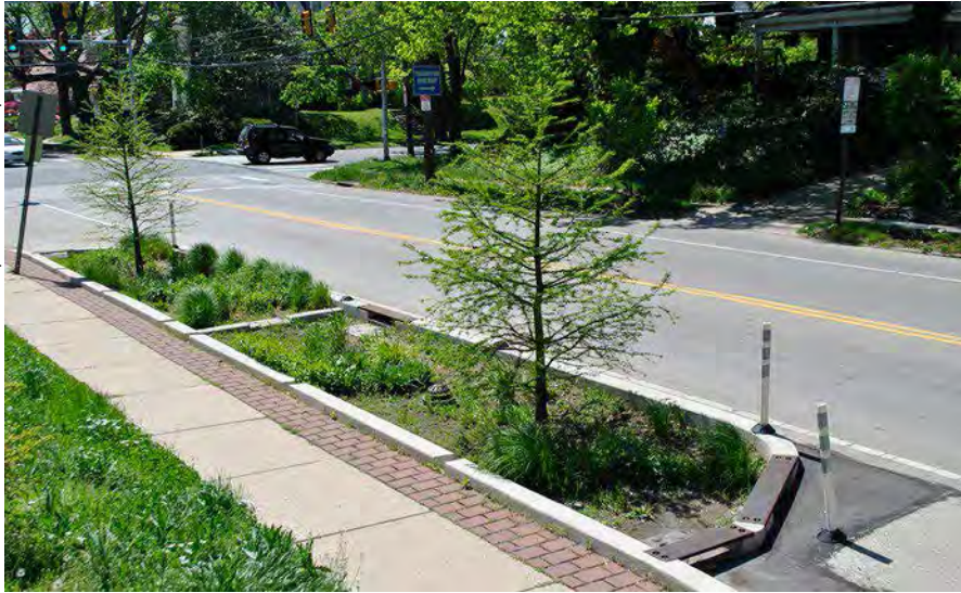
Stormwater curb extension in Philadelphia, PA.
