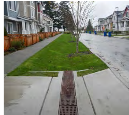
Trench Drain (City of Seattle and MIG/SvR)
