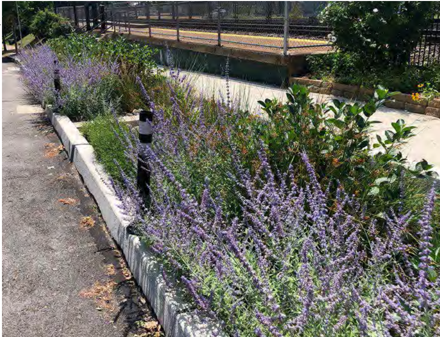
Stormwater curb extension bioretention in Philadelphia, PA.
