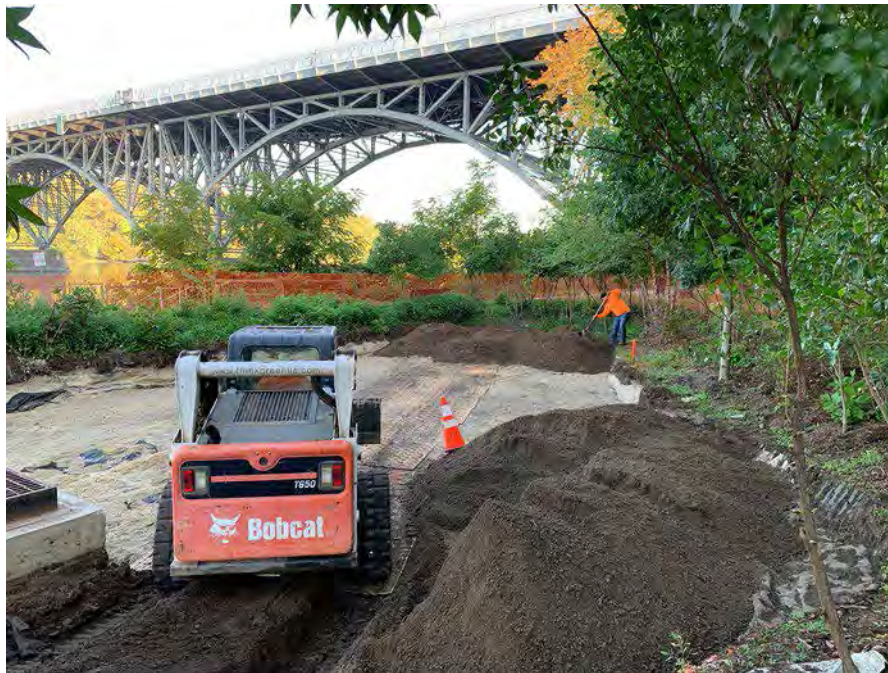
Soilless Soil Initiative project site during construction.
