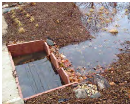
Flagstone Forebay (City of Omaha)
