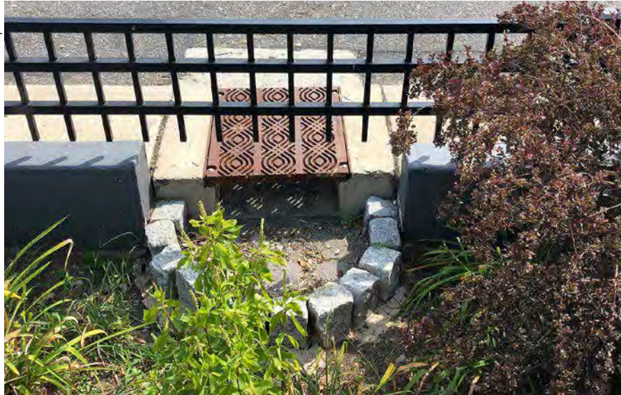
Concrete forebay in New York City, NY.
