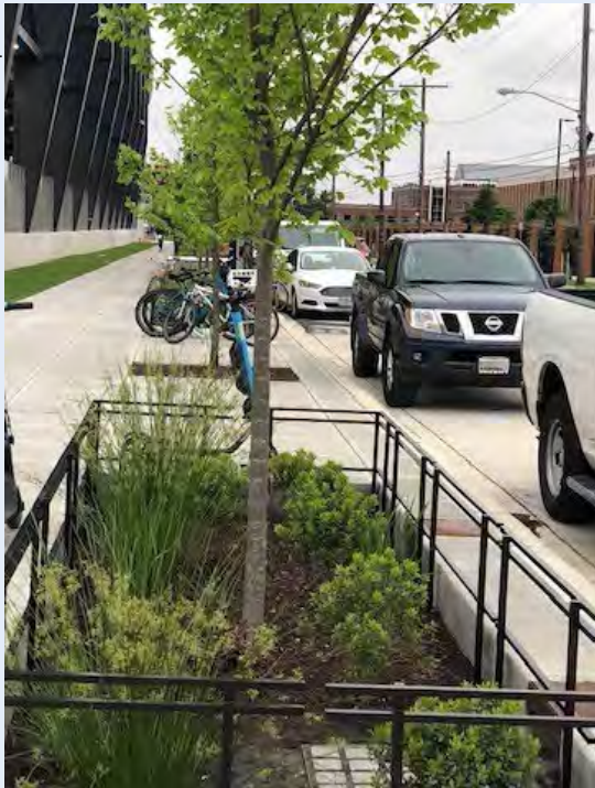
Trees and shrubs are integrated into a series of bioretention facilities in Washington, DC.
