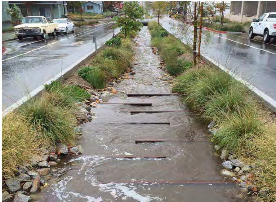
Check dams in a bioretention facility in Paso Robles, CA. These types of in-practice erosion control measures create terraces on the steep grades of sloped streets, prevent erosive flows from entering and damaging bioretention practices, and help control the desired ponding depth. This example also illustrates how check dams can be designed in an artistic manner.
