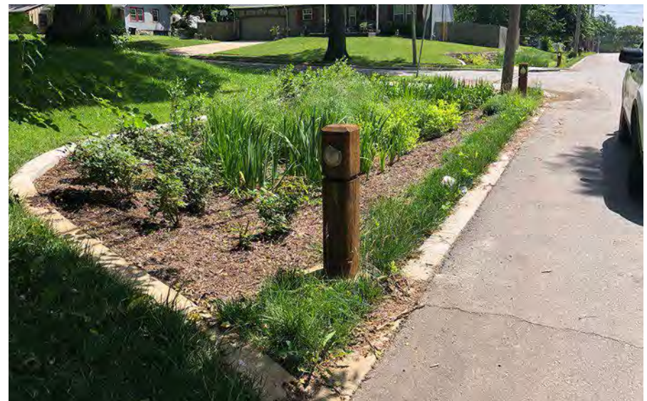
A VFS in a curbsless bioretention facility treats incoming sheet flow in Kansas City, MO.
