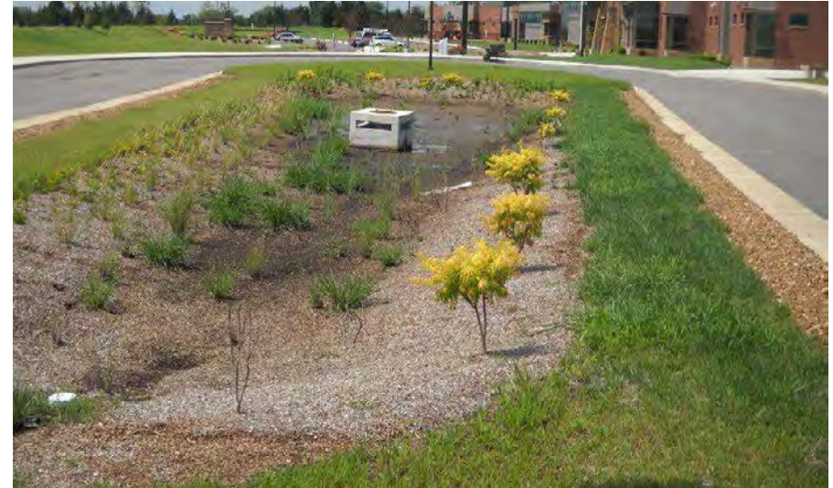
Curbless bioretention with a level spreader and VFS in Omaha, NE.
