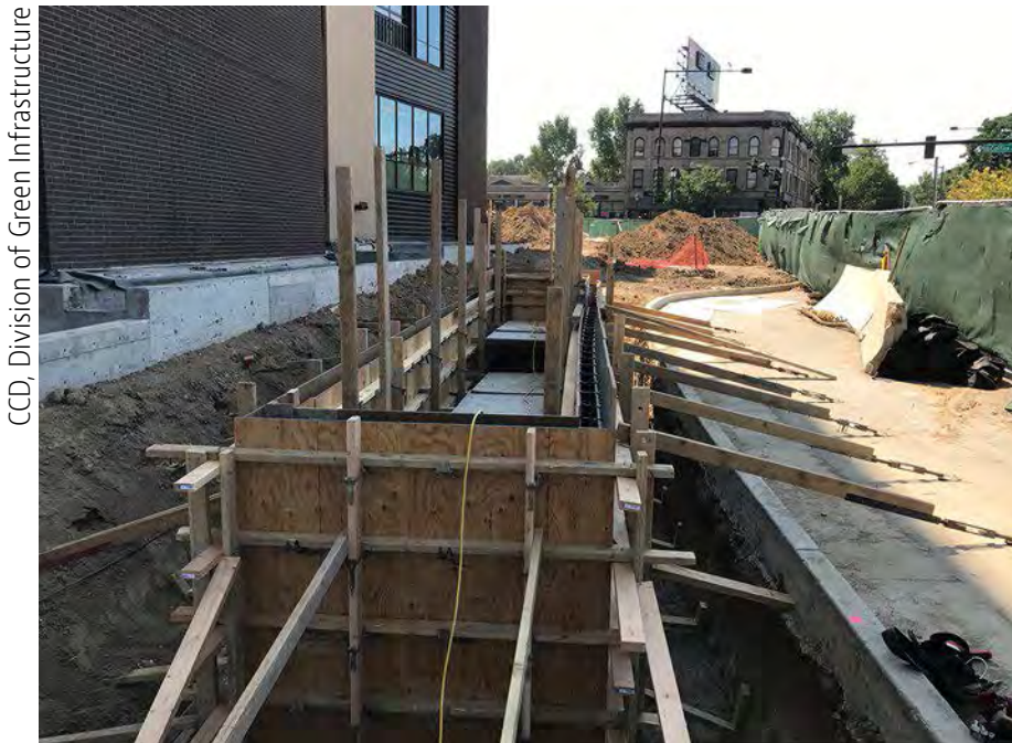
Bioretention under construction in Denver, CO.
