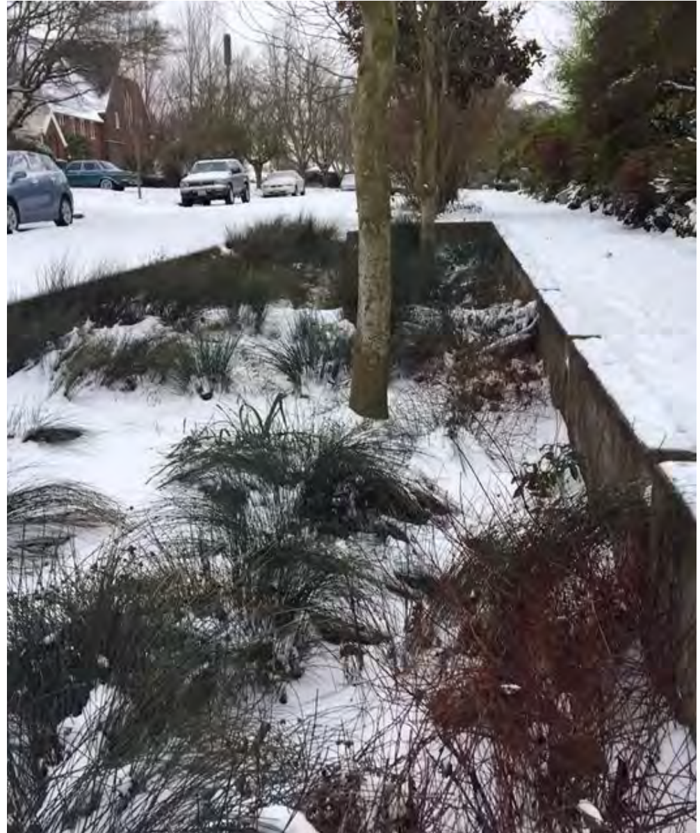
A bioretention facility after a snowfall in Portland, OR.
