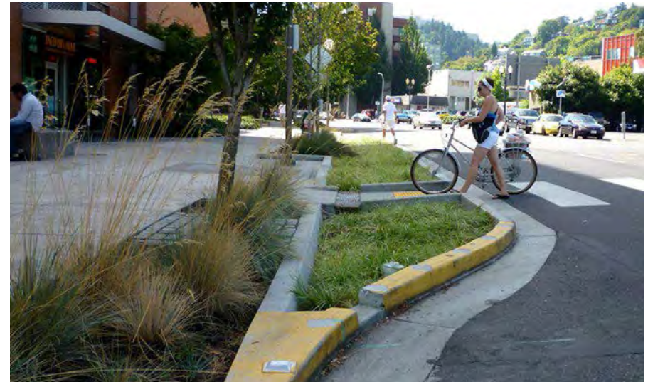
Stormwater curb extension facility that accommodates pedestrian crossing in Hoboken, NJ.
