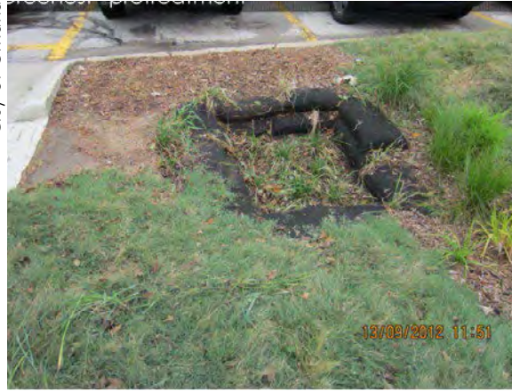
A vegetated bag forebay in Omaha, NE.
