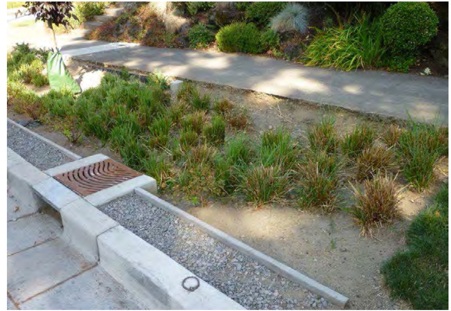
Examples of two step-out zone designs (left, right) in Portland, OR. Concrete is generally preferable over gravel due to weed growth.
