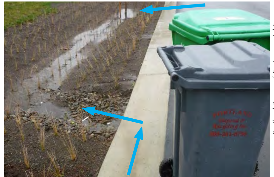
A valley gutter concentrates sheet flow from upstream and can cause localized deposition of debris as it flows into a bioswale in Portland, OR.
