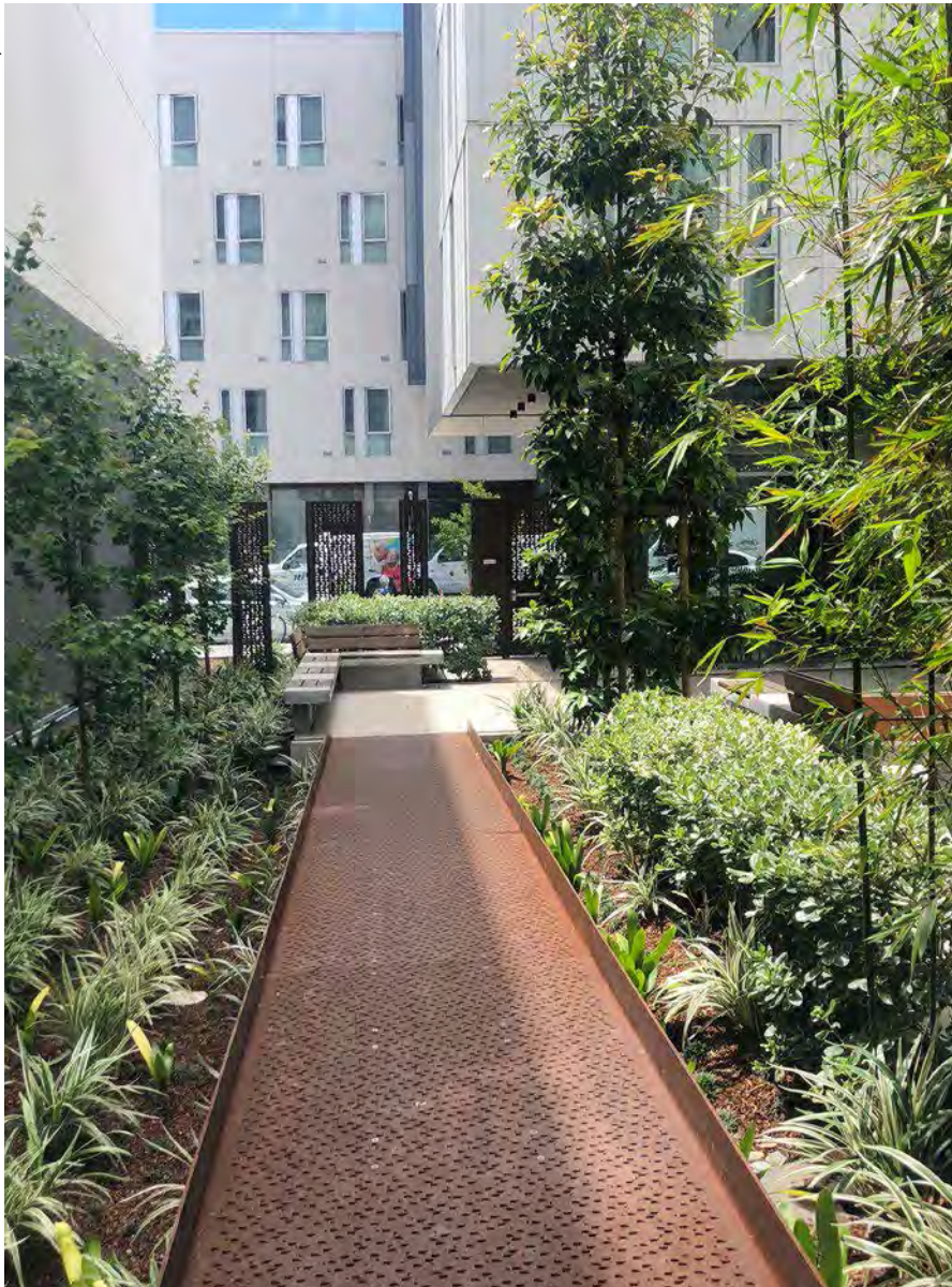
A trench drain crosses a bioretention practice in San Francisco, CA.
