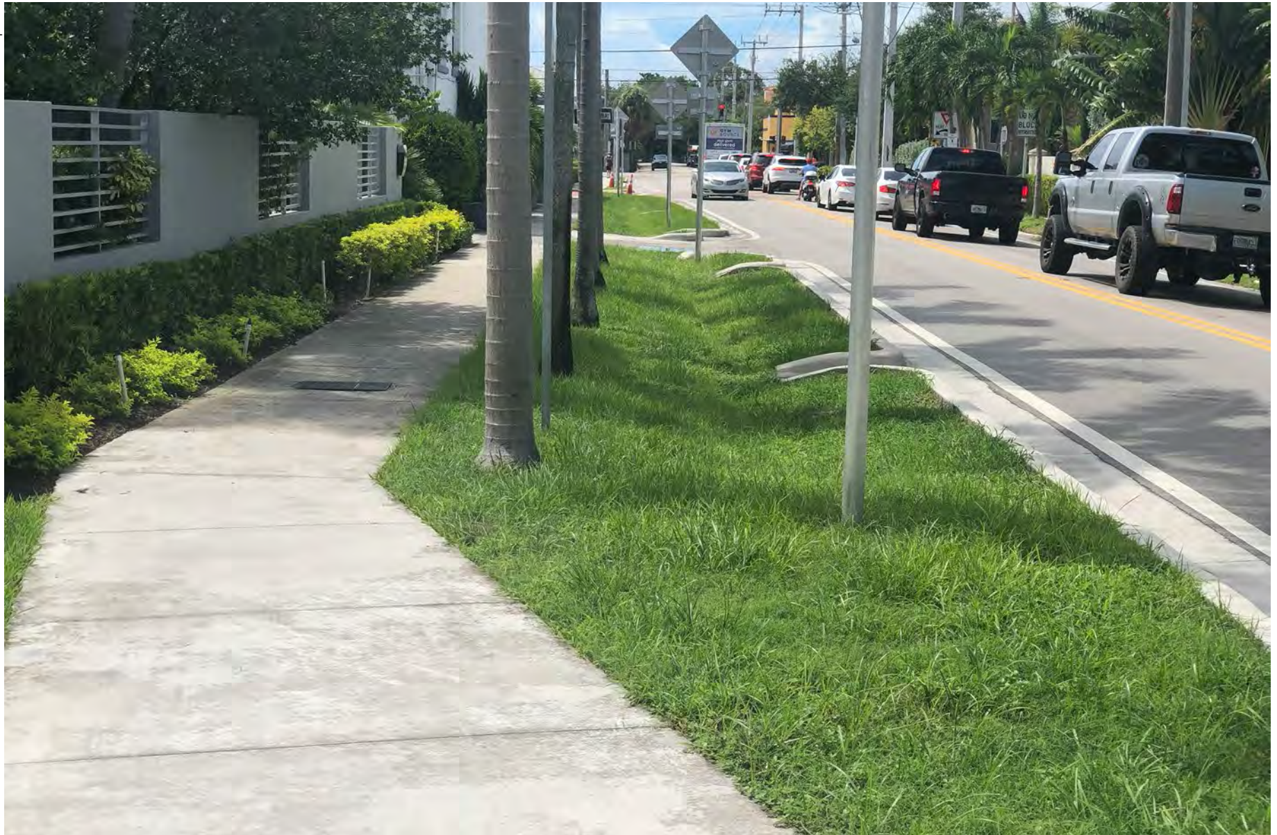
This grassy street-side bioswale is easy to clean and maintain and fits in with the community aesthetic in Fort Lauderdale, FL.
