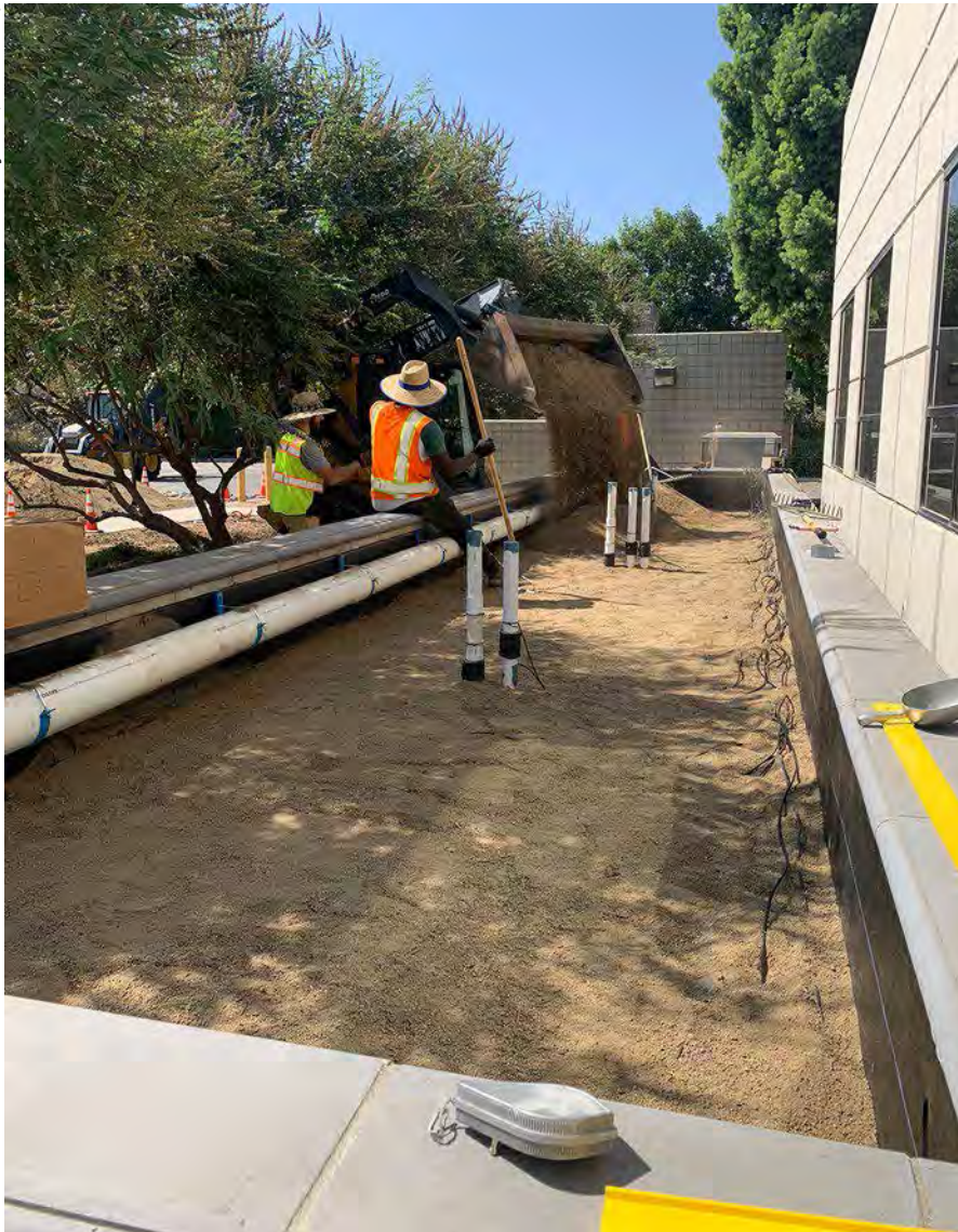
BSM installation for a bioretention planter implemented by the Riverside County Flood Control and Water Conservation District, Riverside, CA.
