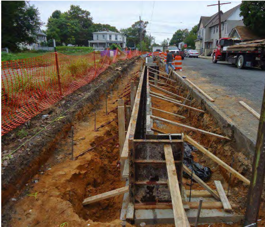
Bioretention under construction in Camden, NJ.
