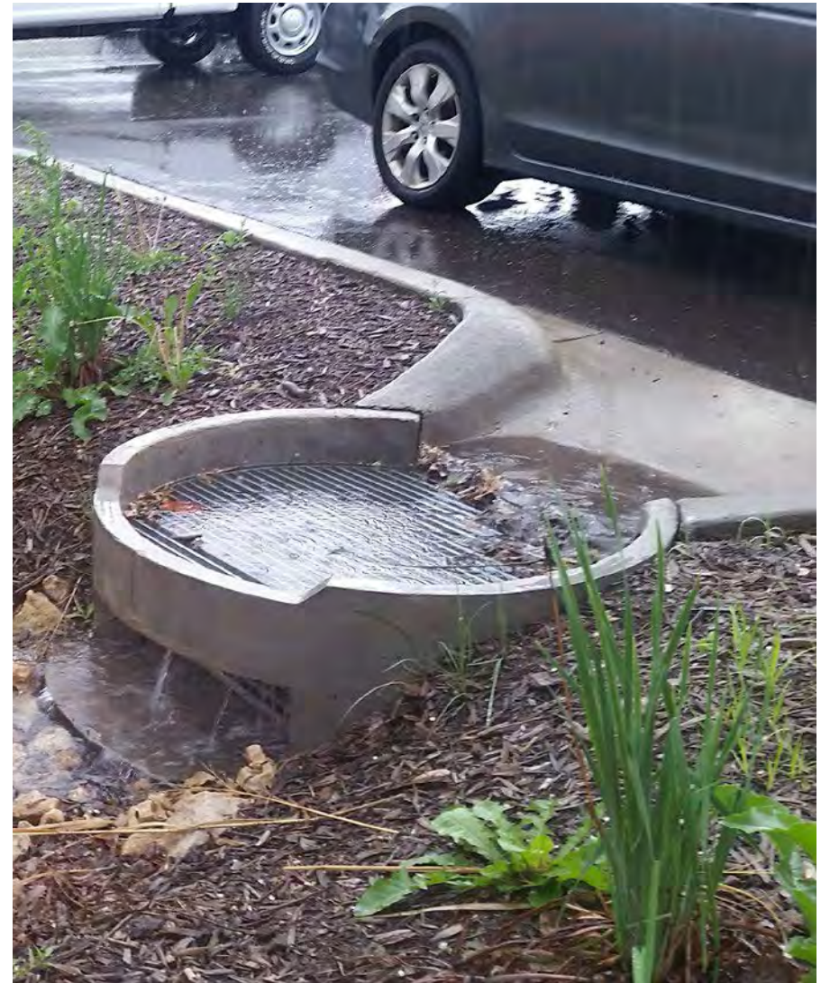
Proprietary inlet sump in Minneapolis, MN.
