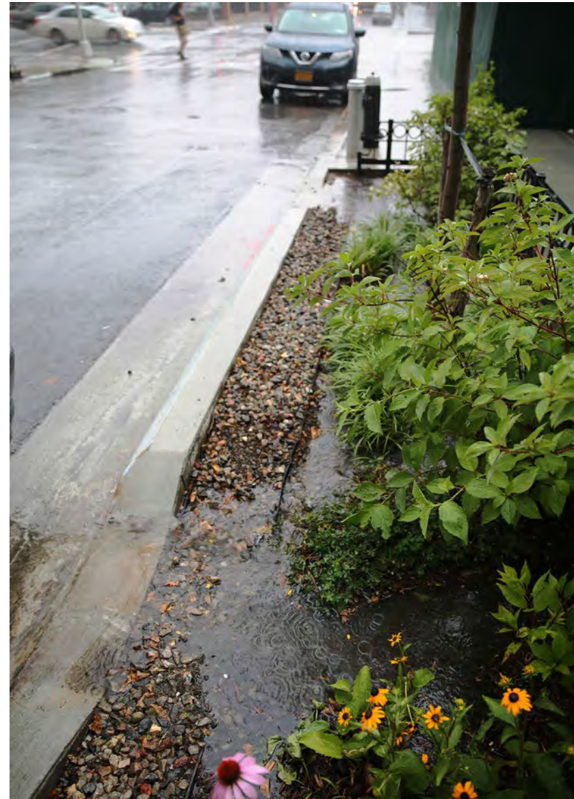
A bioretention practice manages drainage from a street in New York City, NY.
