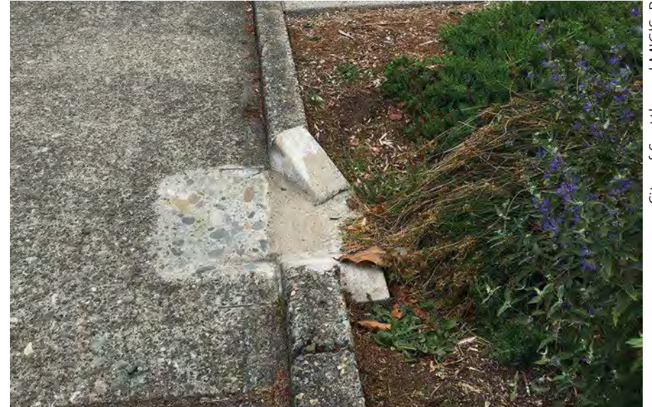
An angled curb cut in Seattle, WA.
