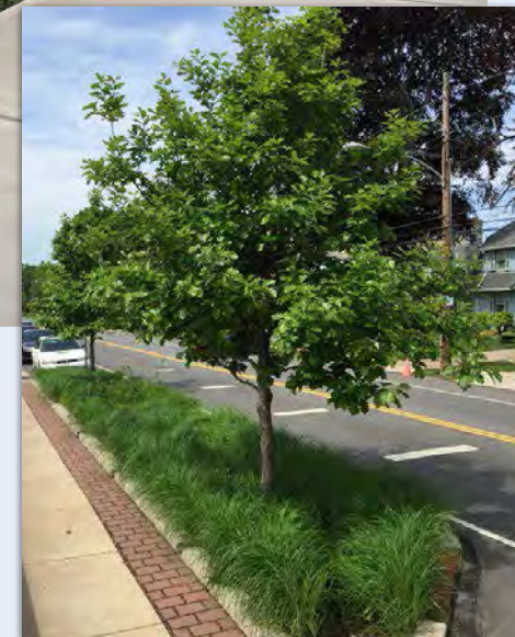
Bioretention facility with trees in Philadelphia, PA.
