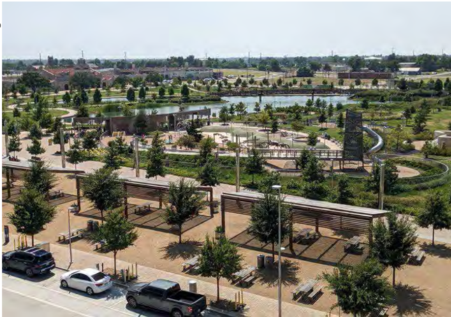
Holistic design incorporates stormwater management and community use in Oklahoma City, OK.
