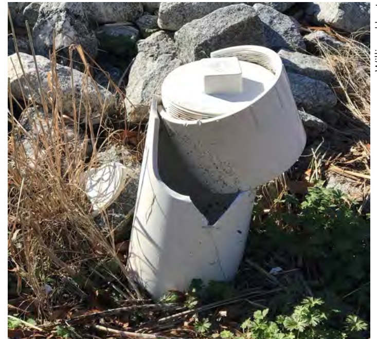
A broken cleanout.
