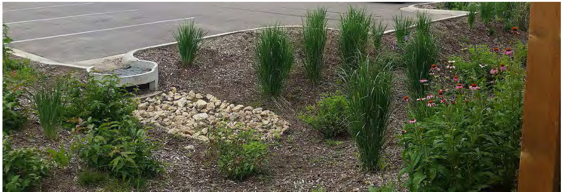
Inlet sump forebay paired with a rock forebay in Minneapolis, MN.
