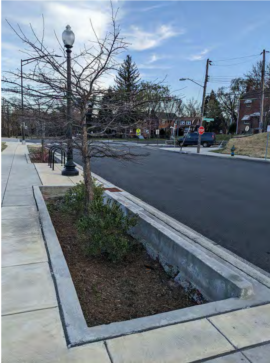
A street-side bioretention planter in Washington, DC.
