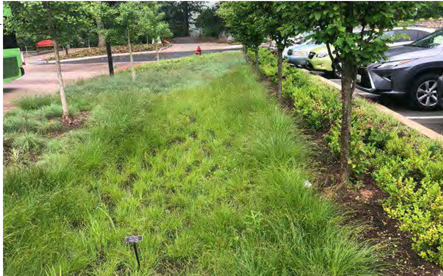
Bioretention with low-height plants in a parking lot in Montgomery County, MD.
