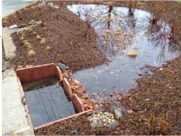
A flagstone forebay in Omaha, NE.
