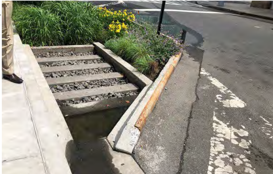
Concrete forebay in New York City, NY.
