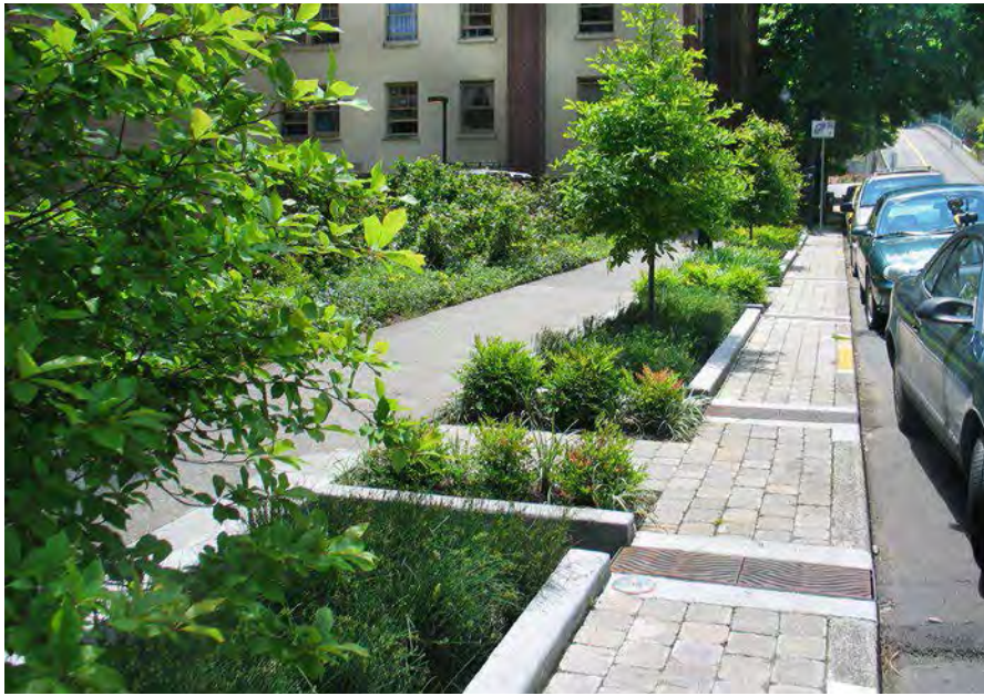
Examples of two step-out zone designs (left, right) in Portland, OR. Concrete is generally preferable over gravel due to weed growth.
