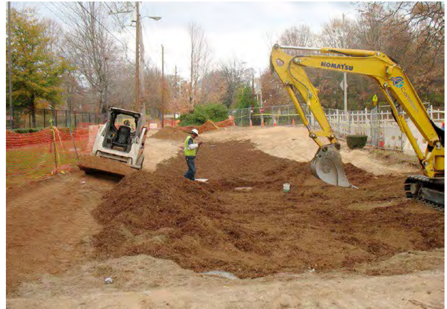
Bioretention facility under construction in Atlanta, GA.
