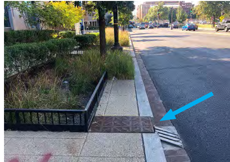
A road is graded toward a bioretention practice in Washington, DC.
