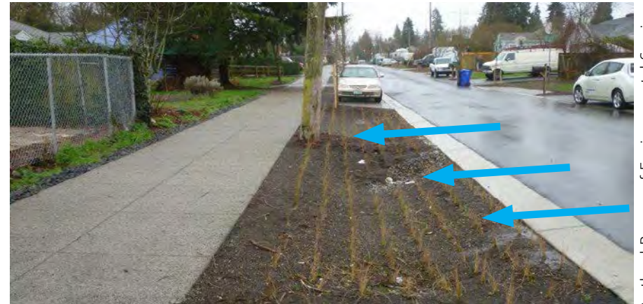
Sheet flow is directed off a residential street by using a gentle slope along the street crown and a curbless gutter (valley gutter) in Portland, OR.
