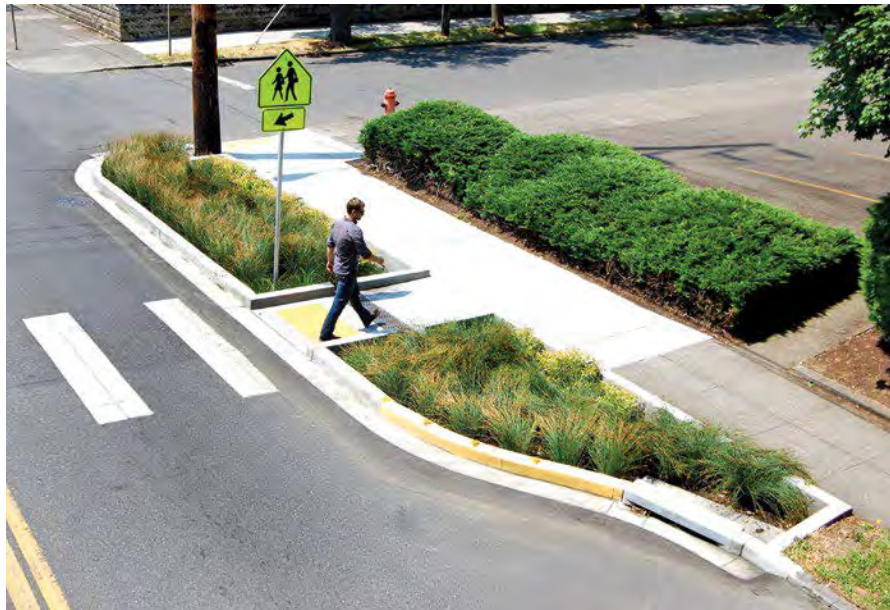
This GSI design treats runoff while guiding pedestrians safely to the crosswalk.
