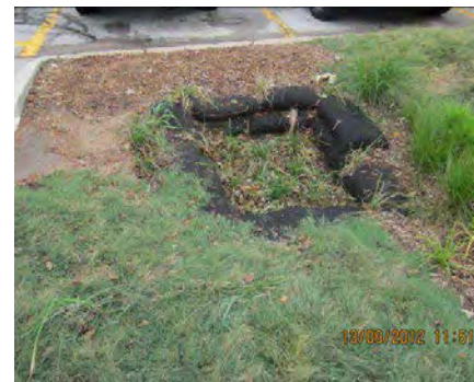
Vegetated Bag Forebay (City of Omaha)
