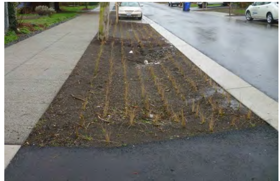
Curbless bioretention with a level spreader in Portland, OR.
