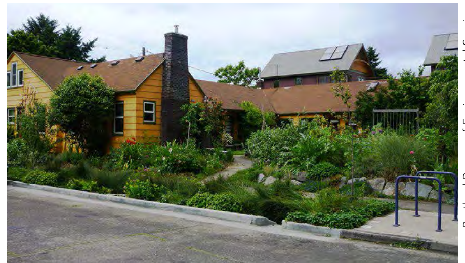
Street-side bioretention in Portland, OR.
