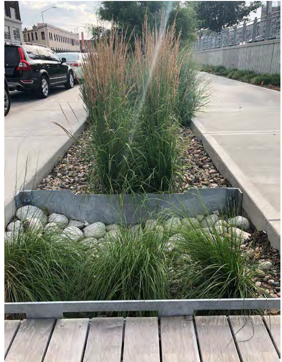
Check dam used for energy dissipation in a bioretention planter box in Kansas City, MO.
