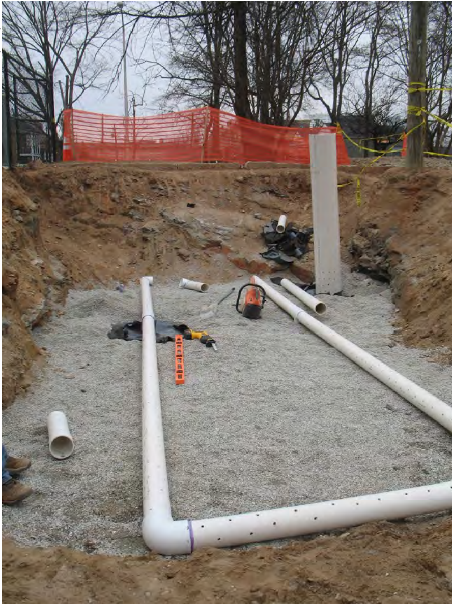
Underdrains being installed in Atlanta, GA.
