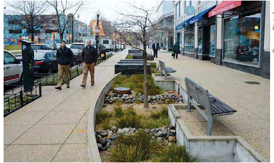
Bioretention with low fencing and walls for safety and benches for pedestrians in Washington, DC.
