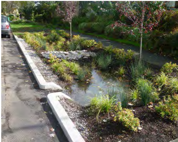
These three bioretention facilities lack proper step-out zones, creating a safety hazard for individuals entering and exiting vehicles. Providing easy access to step-out zones and pathways allow for pedestrian circulation and minimize trampling-related system damage.
