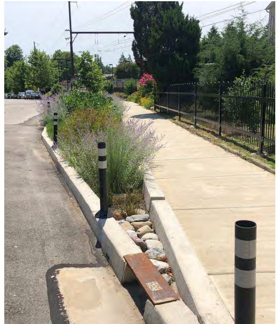
Reflective bollards alert drivers about a stormwater curb extension bumpout in the road in Philadelphia, PA.
