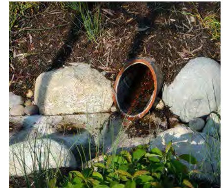
Pipe (City of Seattle and MIG/SvR)
