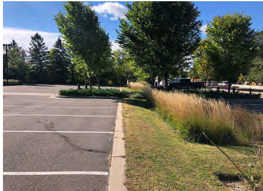
A bioswale includes gentle grades and low-growing vegetation, which fits the parking lot site in Minneapolis, MN.
