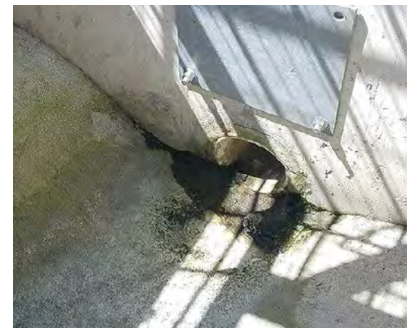
Underdrain outlet in an outlet box.
