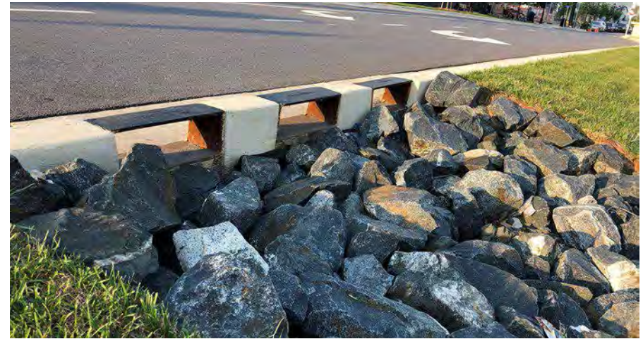
Wheel guards are installed over inlets that are parallel to traffic, such as on this median bioswale in Prince George's County, MD.
