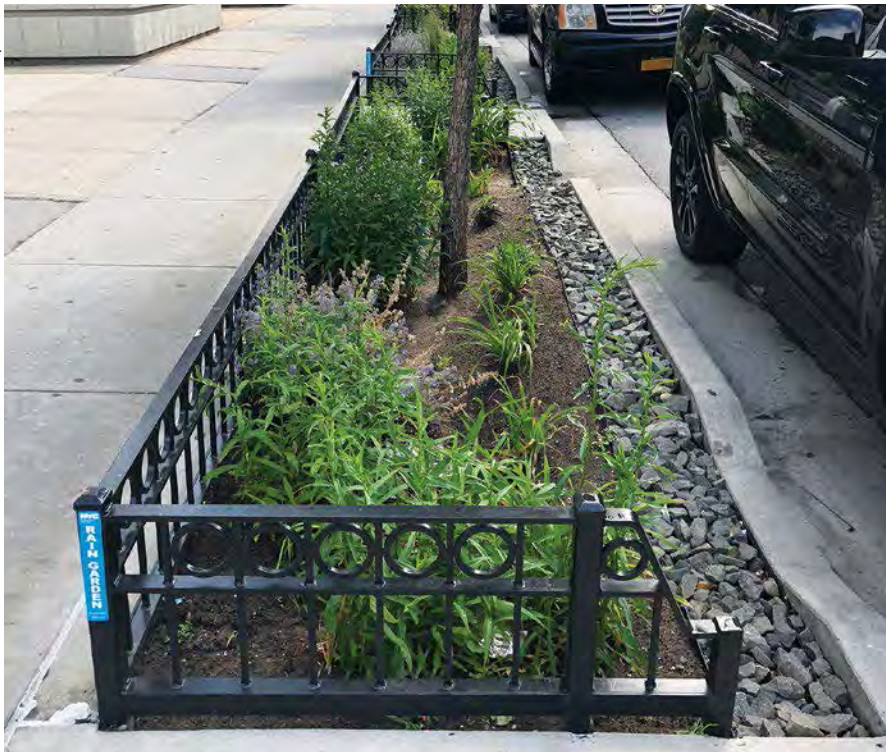
A gravel forebay receives runoff flow and distributes it evenly across this bioretention facility in New York City, NY.
