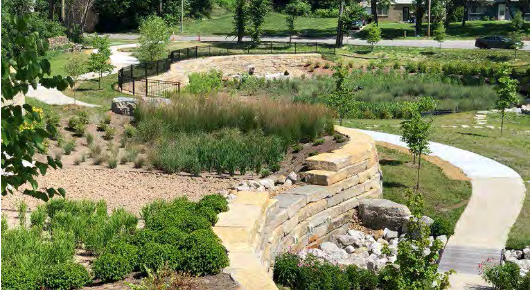
A pedestrian walkway was integrated into the design of this bioretention practice in Kansas City, MO.
