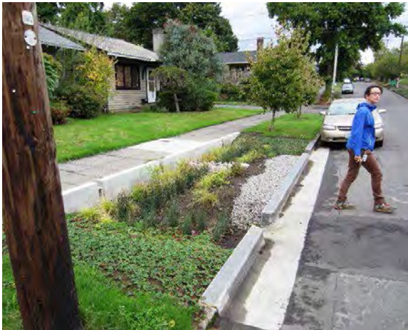
These three bioretention facilities lack proper step-out zones, creating a safety hazard for individuals entering and exiting vehicles. Providing easy access to step-out zones and pathways allow for pedestrian circulation and minimize trampling-related system damage.
