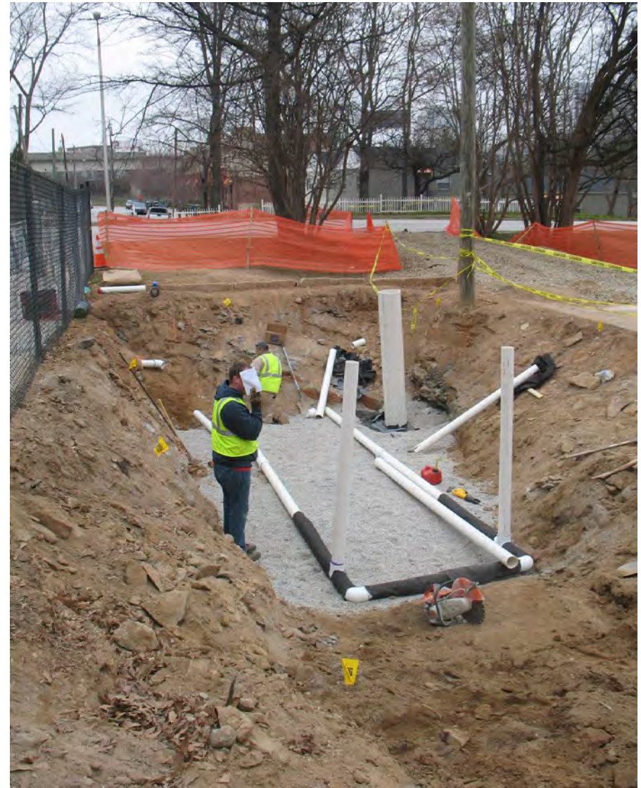
Bioretention under construction in Atlanta, GA.
