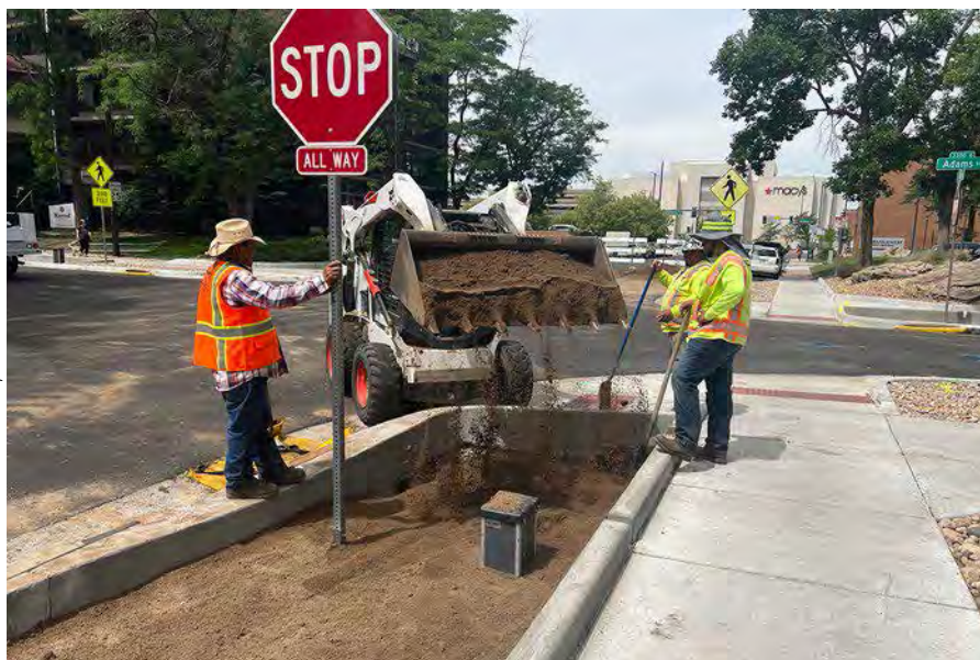
Soil media is visible during facility construction in Denver, CO (left) and Santa Rosa, CA (right).
