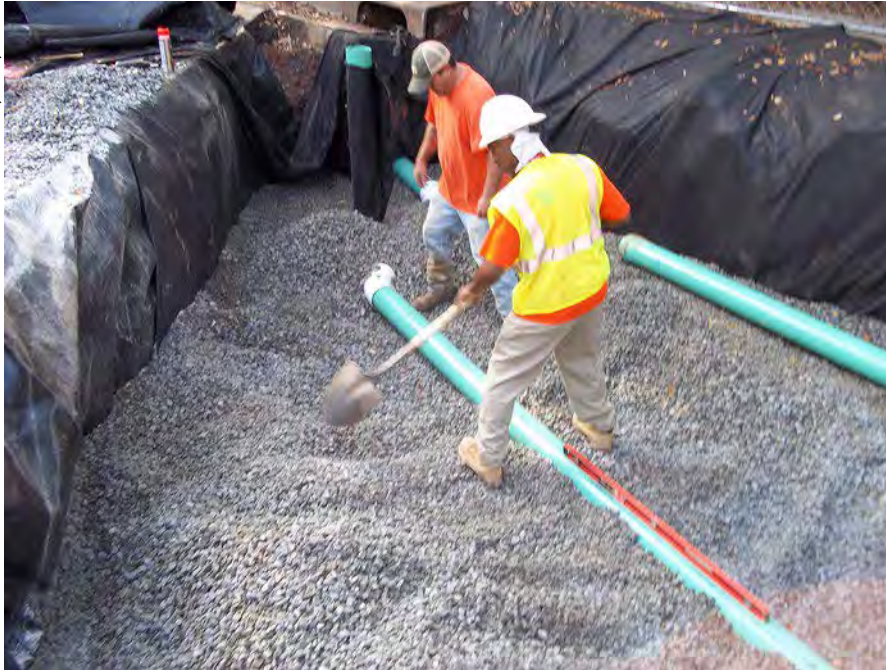
Installing aggregate media in Atlanta, GA.
