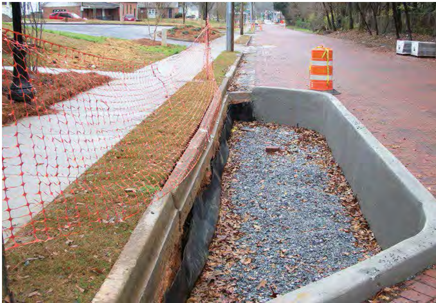
Bioretention under construction in Atlanta, GA.
