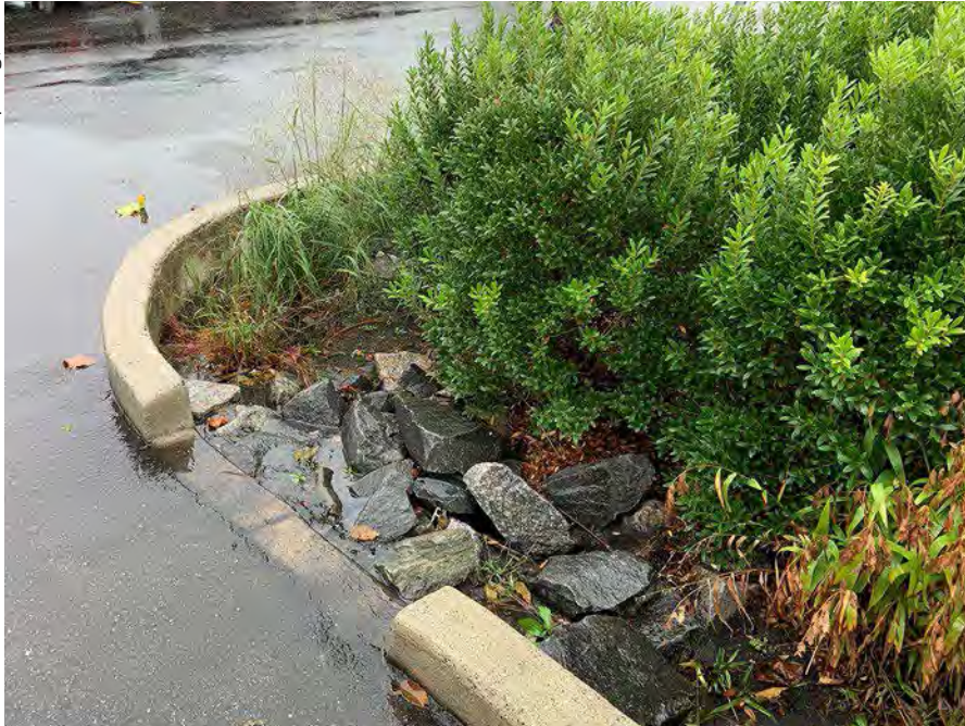
A stone forebay dissipates the energy of incoming flow.
