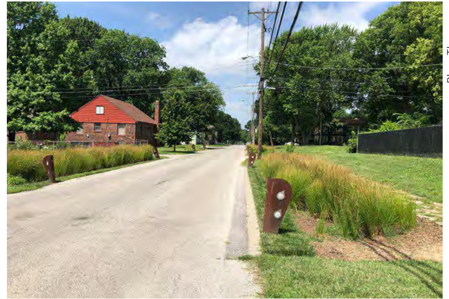
Curbless bioretention in Kansas City, MO.
