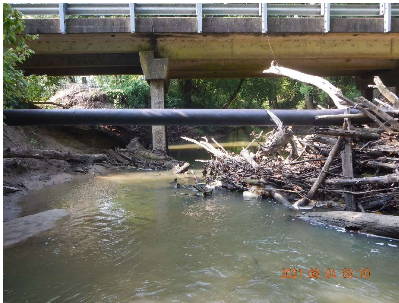
Figure 13: At Station BGEH-46A: Downstream View of Big German Creek (8/4/2021)
