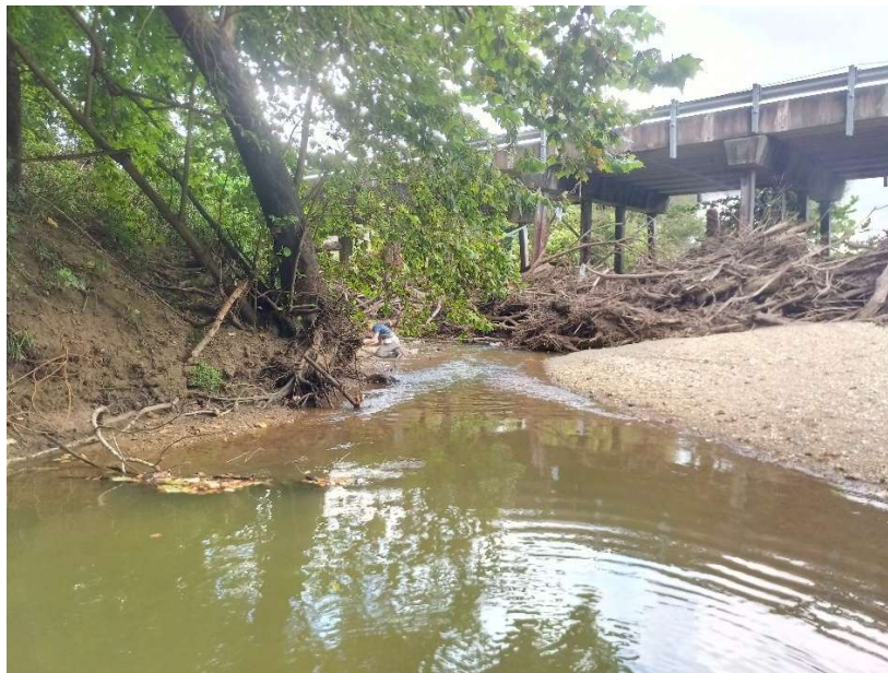
Figure 11. At Station COTH-57C: Downstream View of Cottonwood Creek (8/19/2021)
