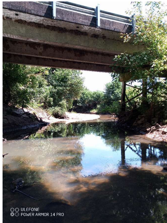
Figure 8. At Station BPRH-44C: Upstream View of Big Prairie Creek (8/12/2024)
