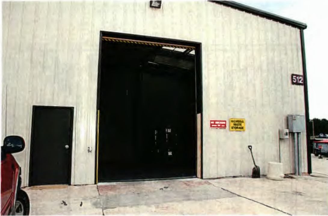
1 FIGURE II B-16 2 Building 512 Exterior
