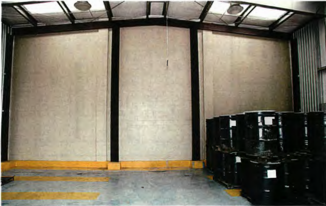
4 FIGURE II B-17 5 Building 512 Interior
