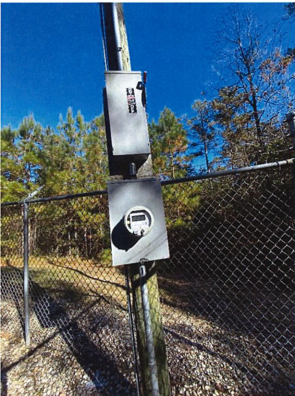
Photo #6 – Hampton Inn Pump Station (Facing East)
