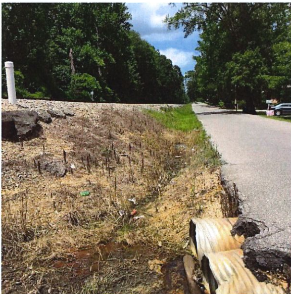
Photo #30 – Warren Street (Facing East)
