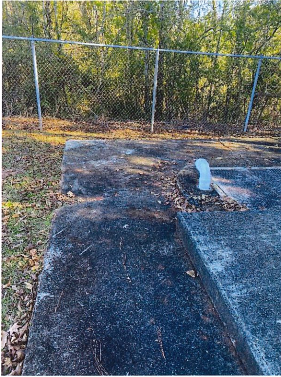
Photo #9 – Windrush Pump Station (Facing East)
