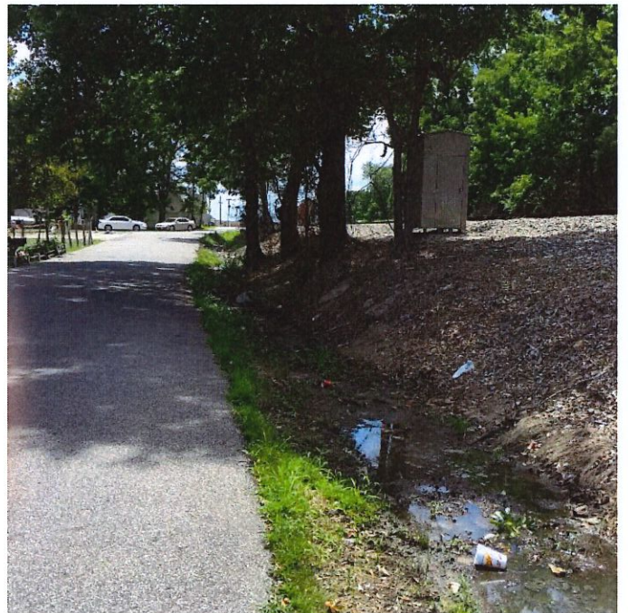
Photo #32 – Warren Street (Facing West)
