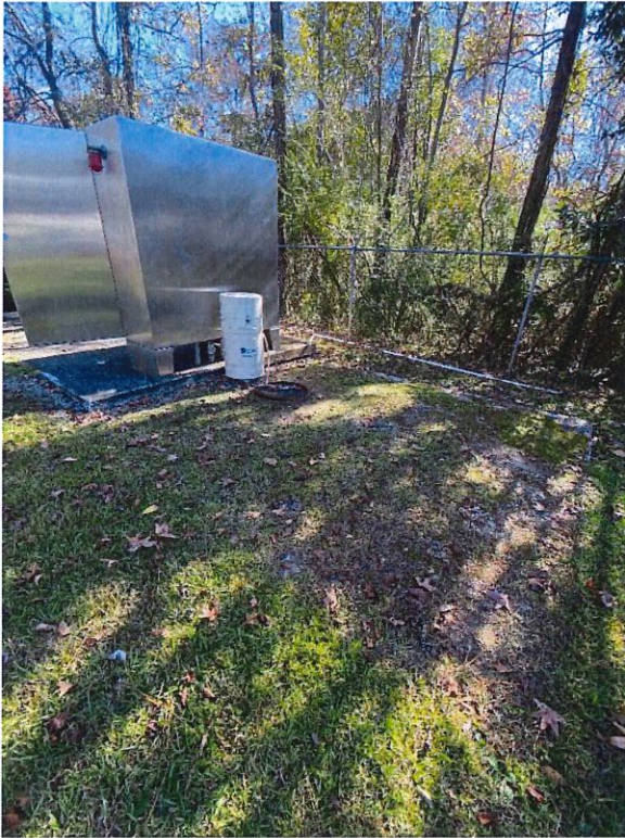
Photo #29 – Jones Drive Pump Station (Facing South)
