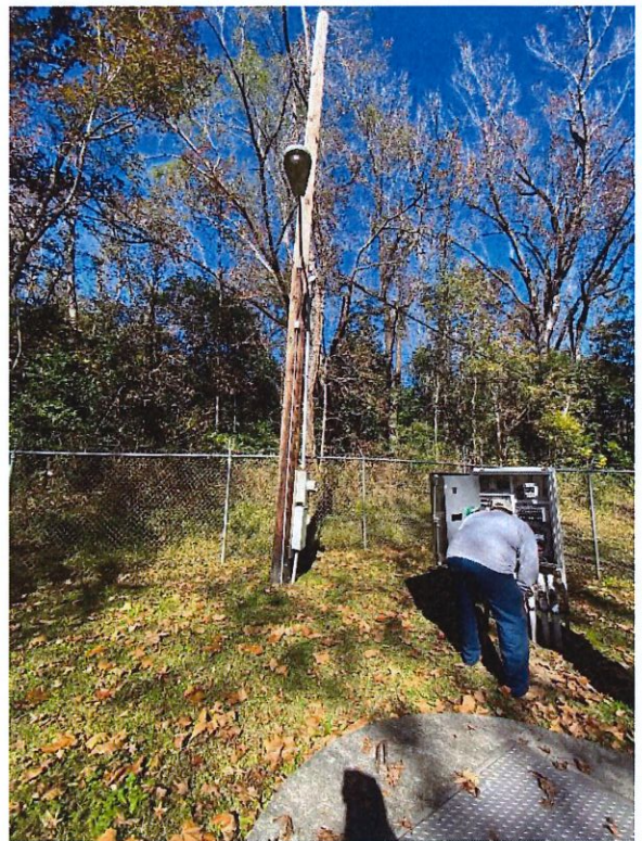
Photo #24 – Davis Pump Station (Facing Northwest)
