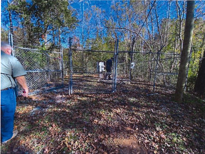
Photo #1– Walmart Pump Station (Facing East)
