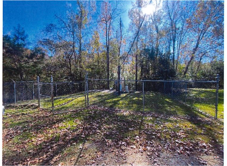
Photo #27 – Jones Drive Pump Station (Facing Southeast)
