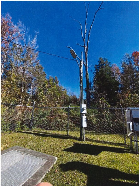
Photo #26 – Willis Pump Station (Facing Northeast)
