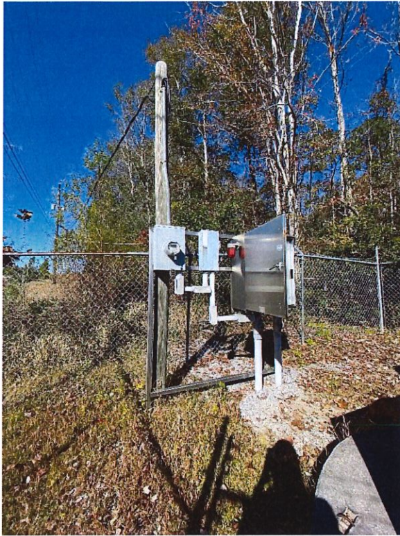
Photo #13 – Napoleon Street Pump Station (Facing North)
