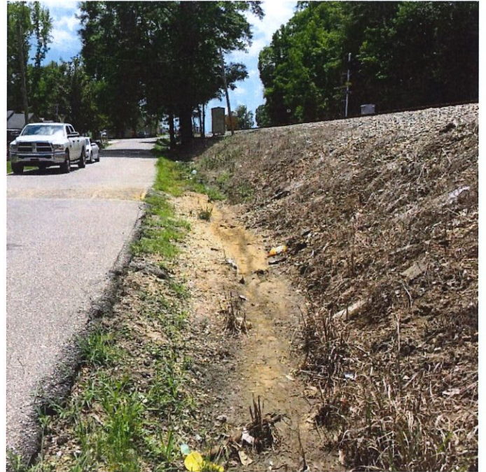
Photo #31 – Warren Street (Facing West)
