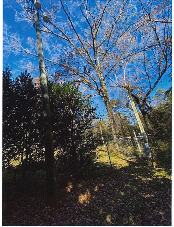
Photo #11 – Glenn Street Pump Station (Facing Northeast)
