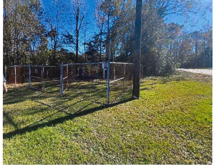
Photo #7 – Windrush Pump Station (Facing South)
