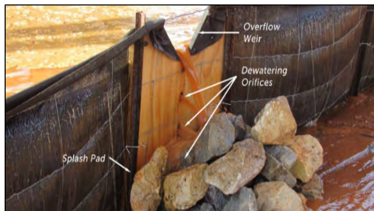
Figure SB-2 Example dewatering board & overflow weir.
