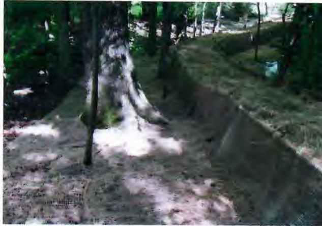
Figure SB-1 Sediment Retention Barrier
