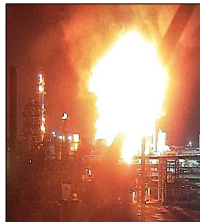
Fired Heater Tube Rupture and fire at Marathon Martinez Renewables
