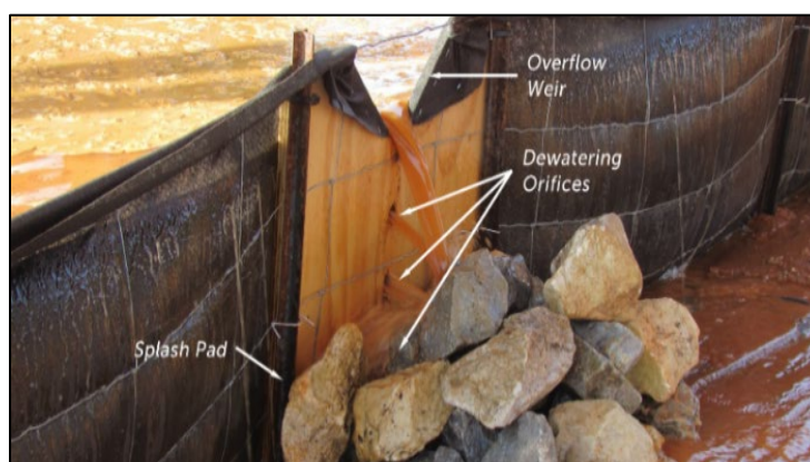
Figure SB-2 Example dewatering board & overflow weir.
