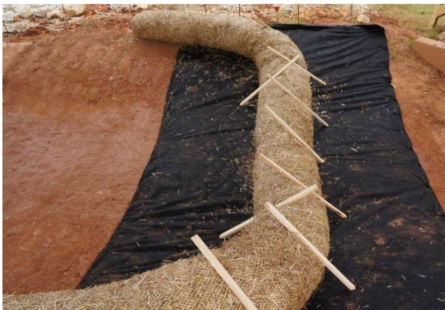
Figure CD-4 Wattle Check Dam (ditch check) (Photo courtesy of Auburn University Stormwater Research Facility)
