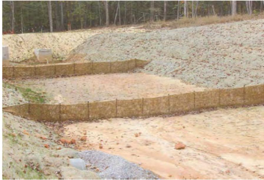
**Figure SBN-2 Example of porous baffle made of 700 g/m<sup>2</sup> coir erosion blanket as viewed from the inlet.** (North Carolina Erosion and Sediment Control Planning and Design Manual.)
