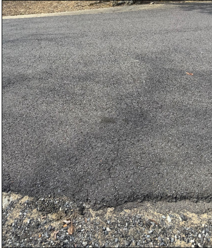
Figure 17. Second Cracked Area Observed in 2025
