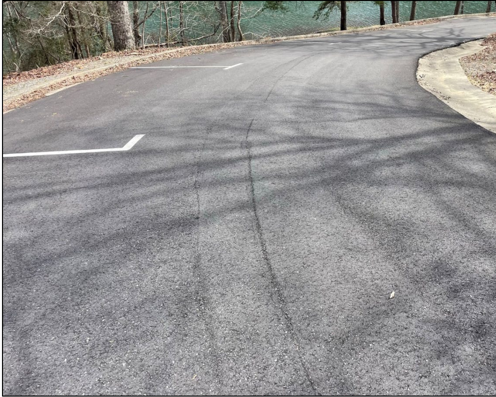
Figure 18. Roller Marks Observed at Desoto Falls Site
