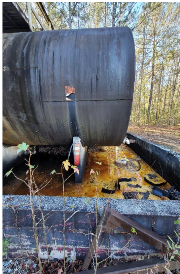
An accumulation of approximately 2 inches of yellowish-orange oil/petroleum/cleaning fluids
