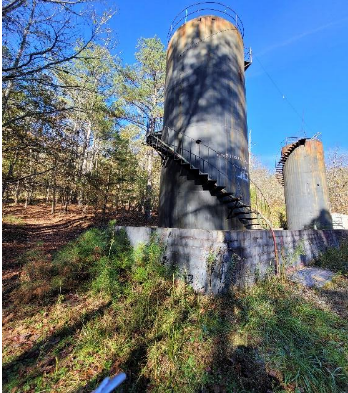
Tank Farm #2- Two vertical tanks within secondary containment
