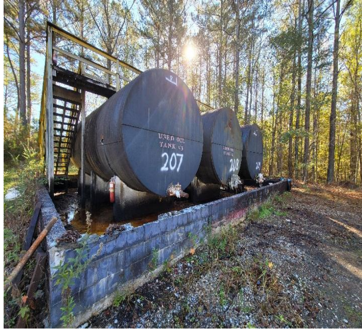
Tank Farm #1- Three horizontal tanks within secondary containment
