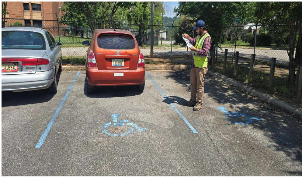
Photo: Photo of existing conditions at Remedial Area 4.
