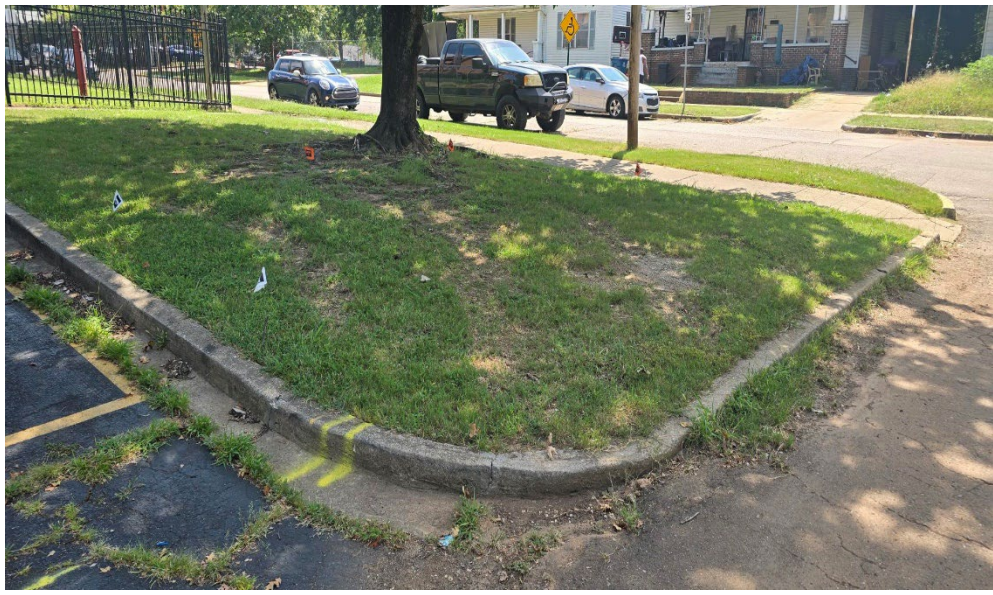
Photo: Photo of existing conditions at Remedial Area 2.
