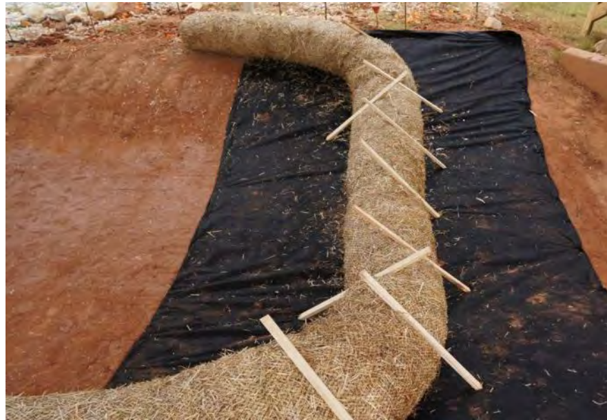
Figure CD-4 Wattle Check Dam (ditch check)
