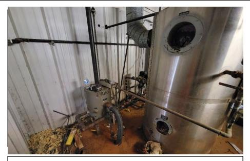
Photograph 5: Boiler used for steam and associated drain hose.
