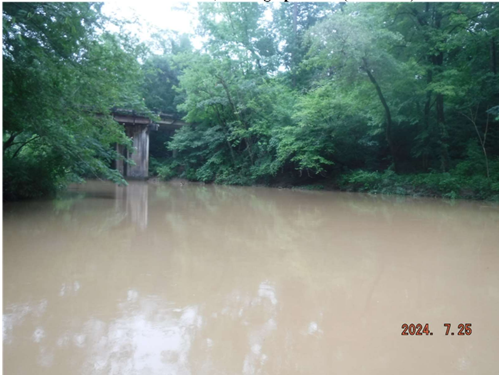
At station FM CJ-6, looking upstream (7/25/2024)
