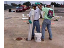
Figure 3. Canister filled with ORC Filter Socks being lowered into treatment well
