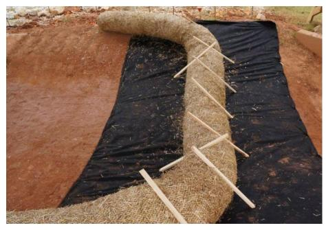
Figure CD-4 Wattle Check Dam (ditch check)
