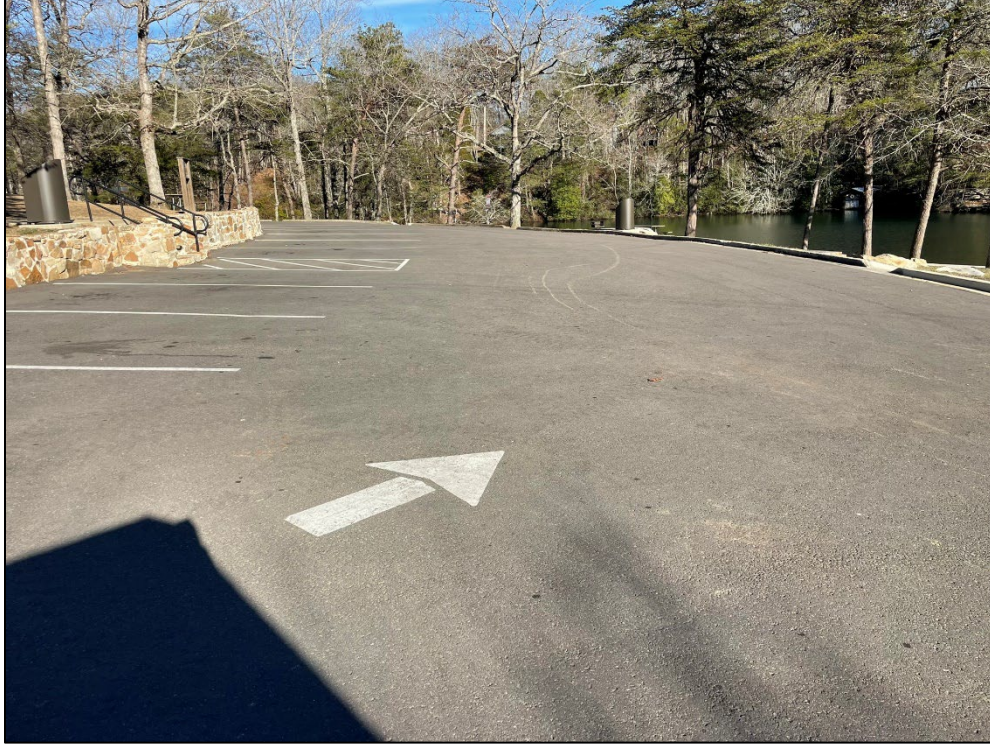
Figure 3 Pavement Example at Desoto Falls Site in 2024
