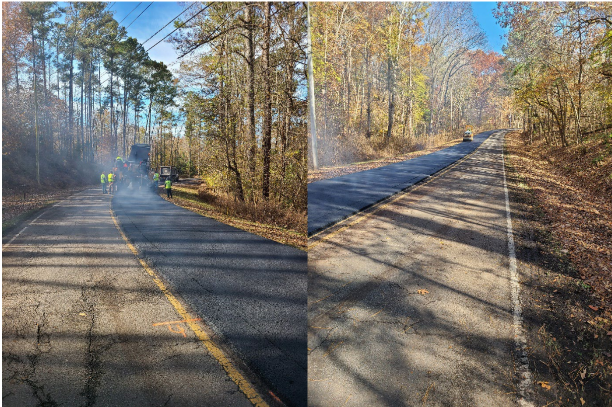
Figure 2. Paving Site in Guntersville State Park
