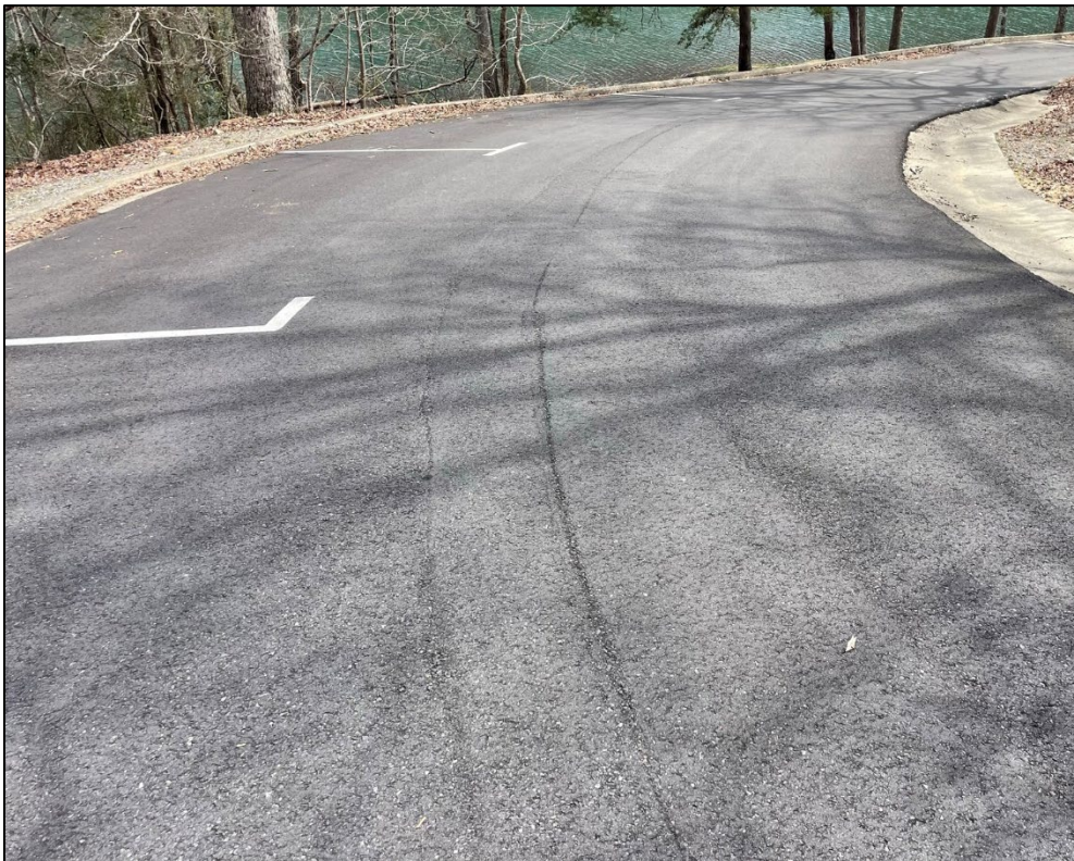
Figure 12. Roller Marks Observed at Desoto Falls Site
