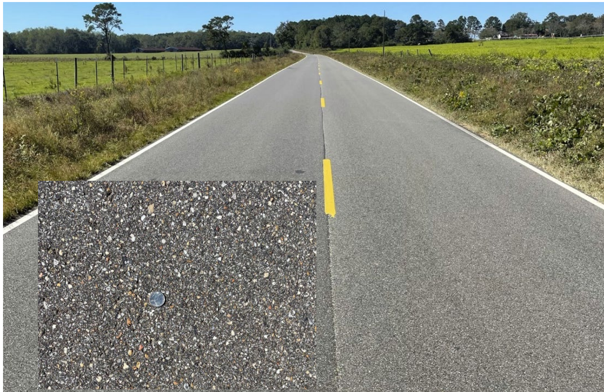
Figure 2 Control Superpave Mix (401) at 12-month Inspection.
