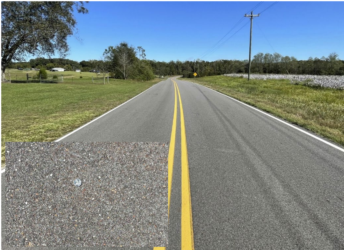
Figure 5 Rubber BMD Mix at 12-month Inspection.
