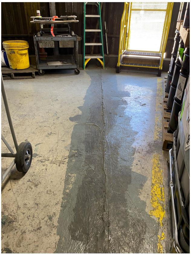
Building 1: Crack at building joint.
