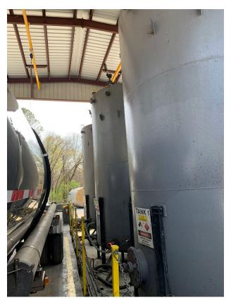
Photo #16: Area between truck pad and tank farm showing aboveground piping and spill containment.
