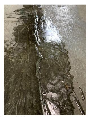
Photo #2: Building #1: Close-up of joint repair.
