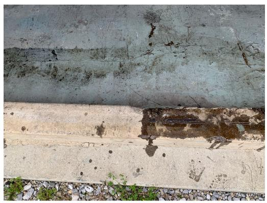
Photo #3: Repair of small cracks in curb at Building #2.
