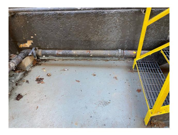
Tank Farm North Wall: Crack in slab at base of wall.
