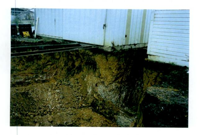
Photograph #8 - Excavation of Former Tank Area. Note the delineation of yellow clay and the white mottled clay.
