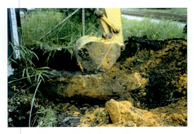
Photograph #4 - Excavation of Tank
