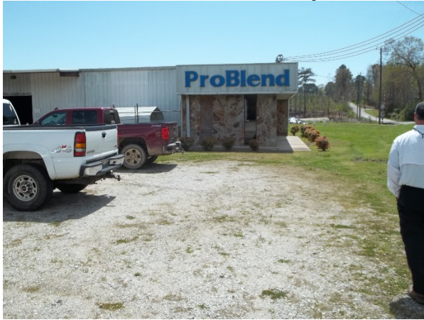
Former ProBlend Facility
