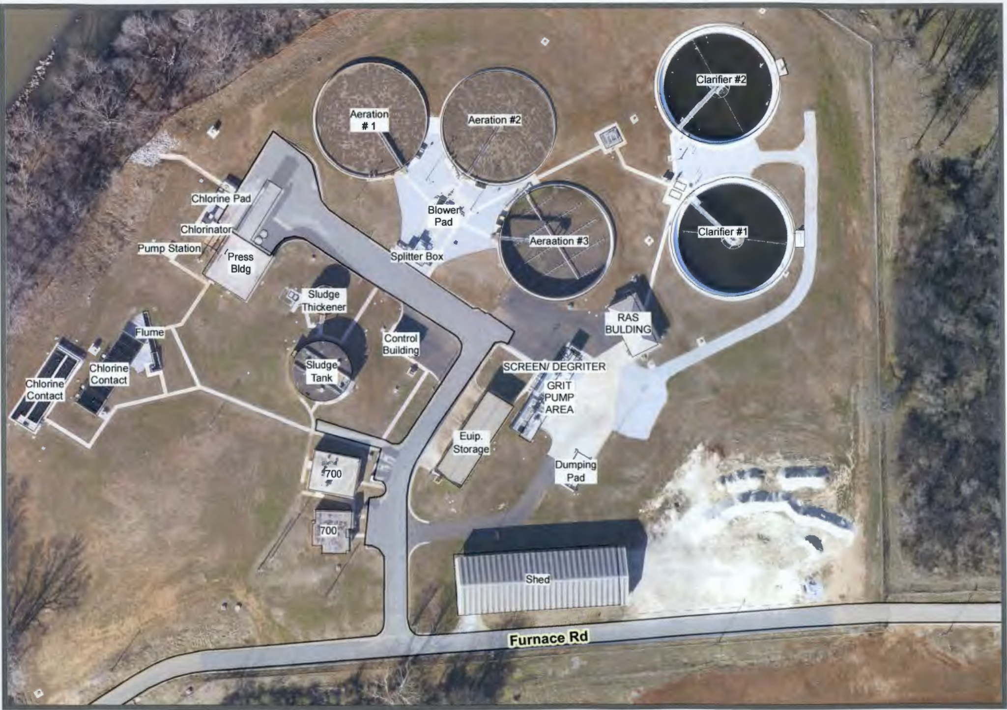
Sheffield Wastewater Treatment Plant
