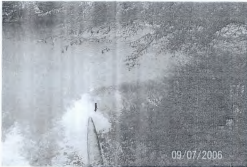
NGC outfall pipe at Choccolocco Creek Talladega County, dwt
