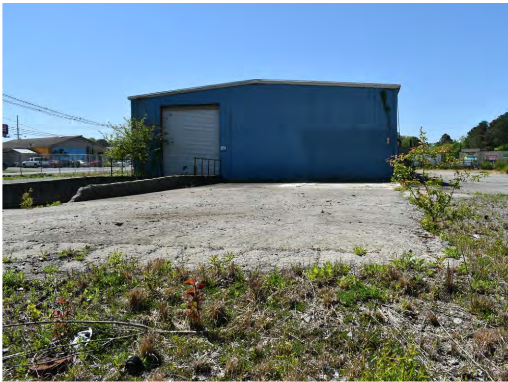
Photo No. 17: Additional view of the north end of the building.
