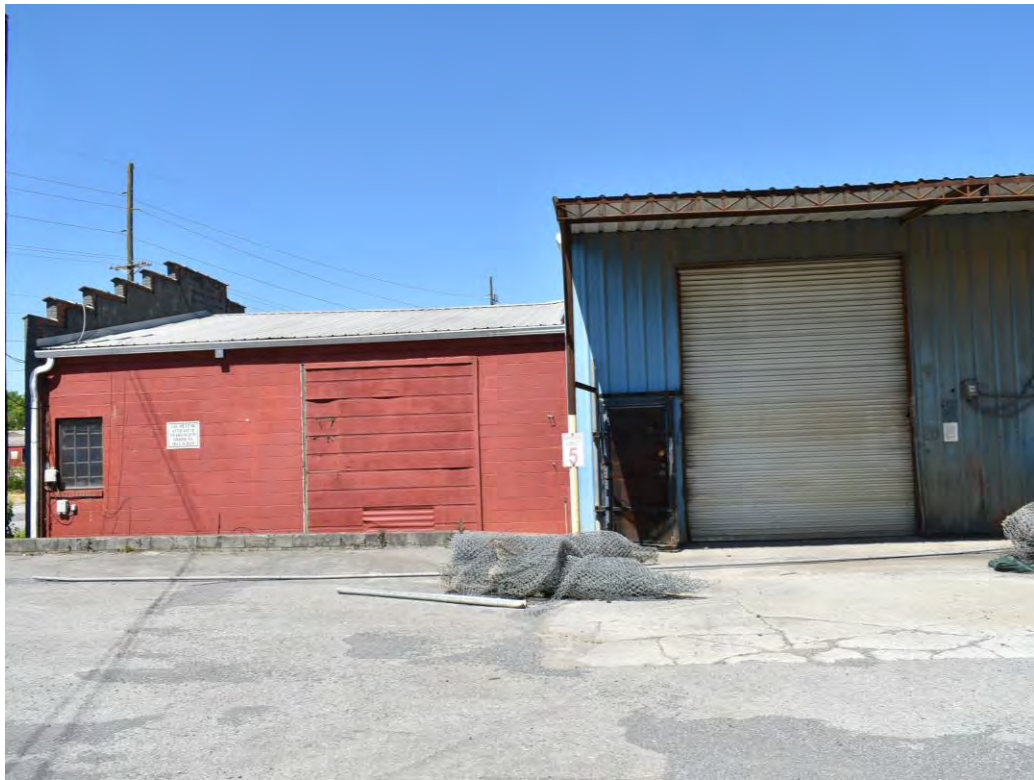
Photo No. 7: View of the southeast portion of the structure previously used as a salvage business.
