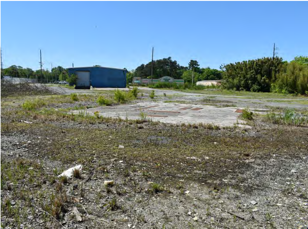
Photo No. 22: Concrete pad in the north-central portion of the subject property.
