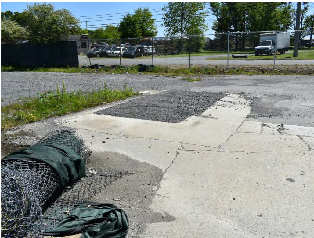
Photo No. 9: View east from the central exterior of the building.
