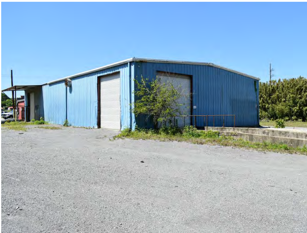
Photo No. 15: View of the northeast portion of the structure.
