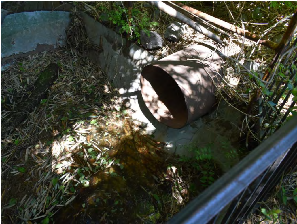
Photo No. 31: Stormwater discharge pipe into the basin.
