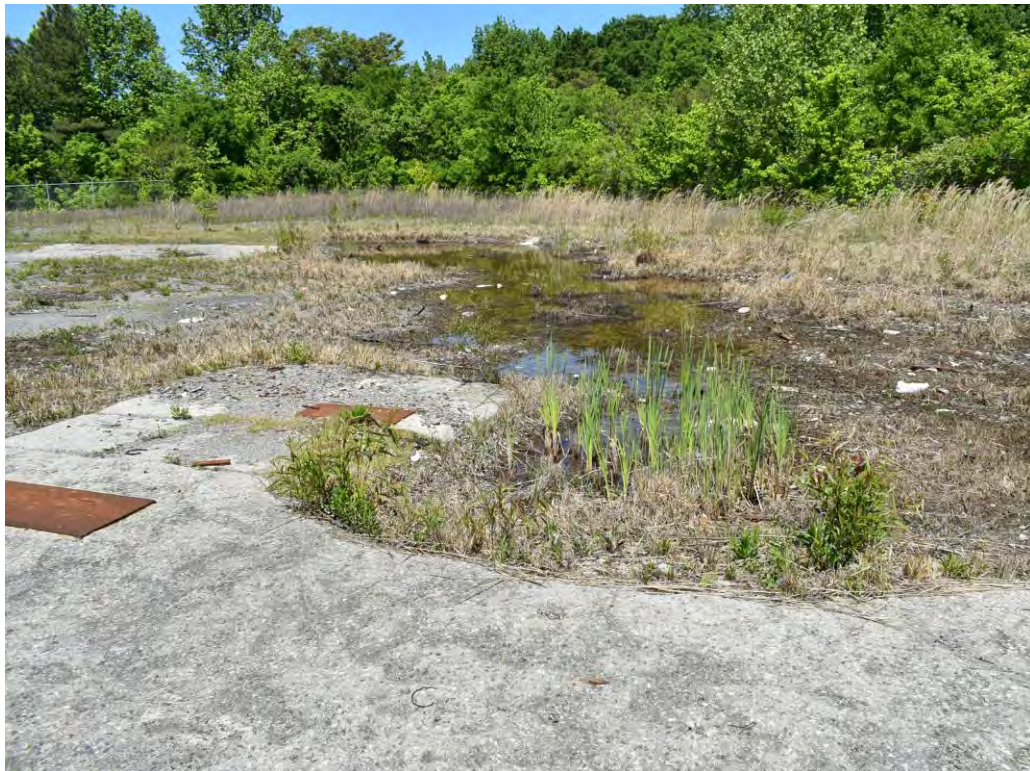
Photo No. 24: View west from the concrete pad.
