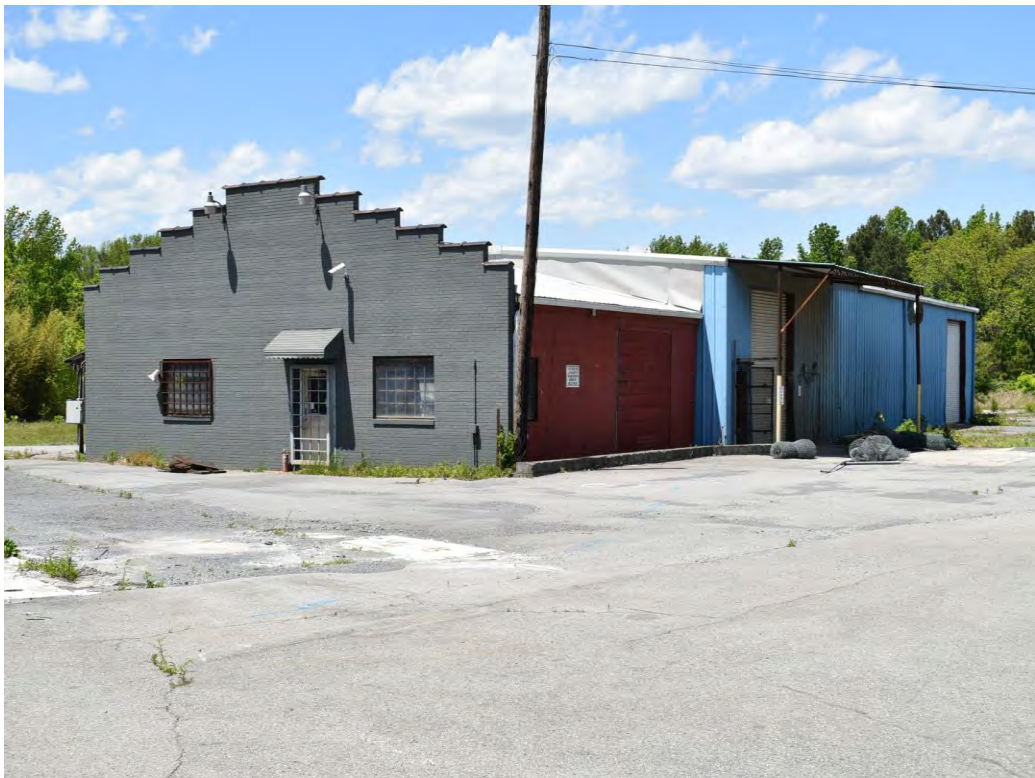
Photo No. 1: Vacant commercial structure at 500 Mathis Mill Road in Albertville, Alabama
