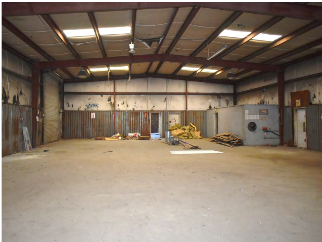
Photo No. 45: View south from the north portion of the warehouse.
