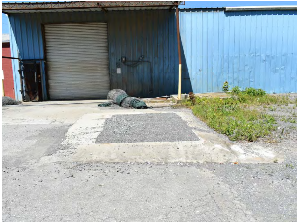
Photo No. 8: Decommissioned scale on the east-central exterior of the structure.
