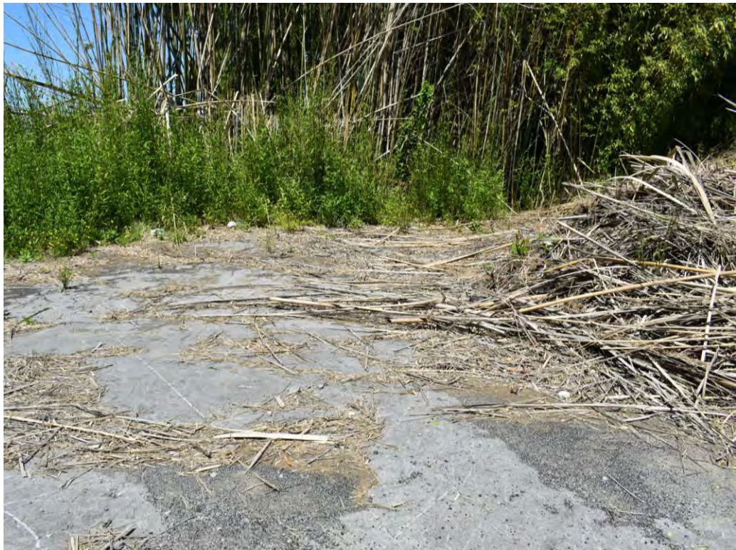
Photo No. 33: View west of the southwest boundary of the subject property.
