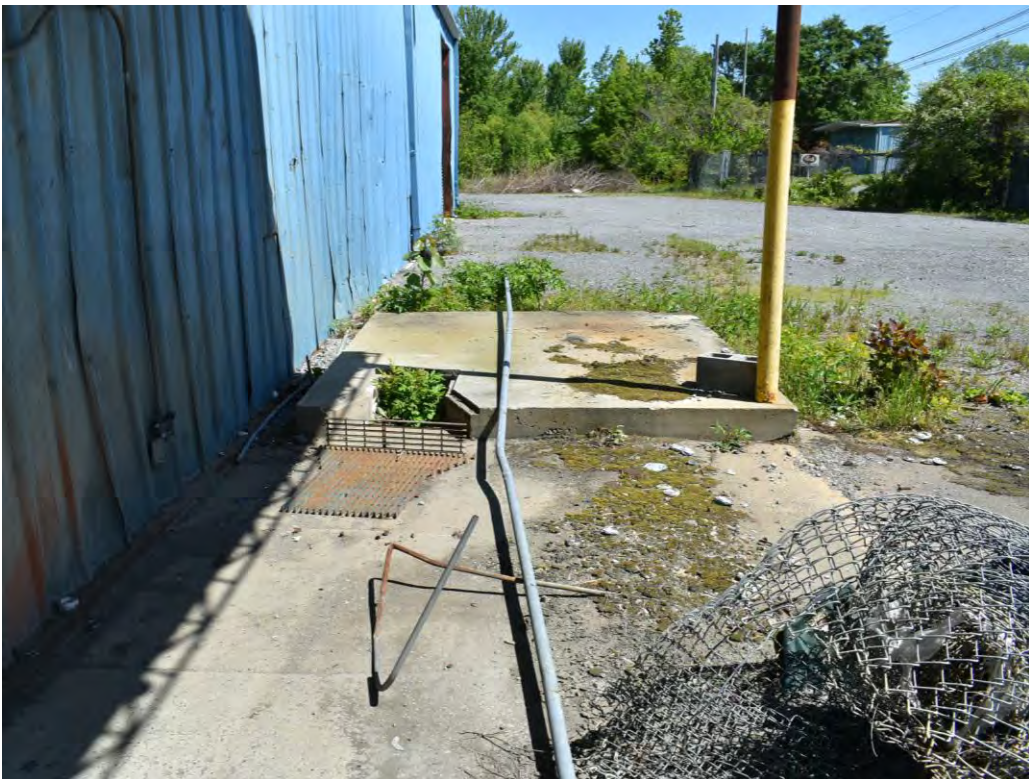
Photo No. 10: View north along the east side of the structure.
