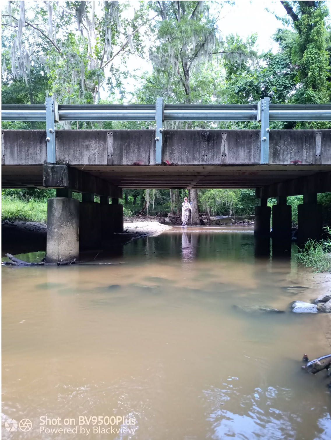
Photo 7-2 Bughall Creek at BGHM-1 (Bullock County Road 177), Looking Upstream
