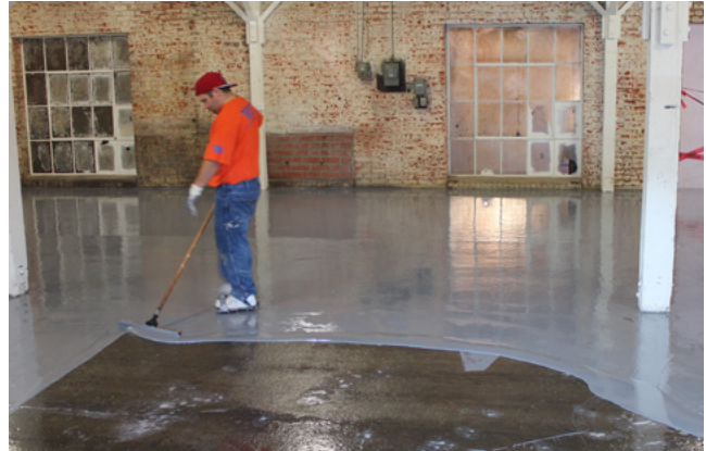
Application of Retro-Coat SEALANT to a 20 mil total thickness
