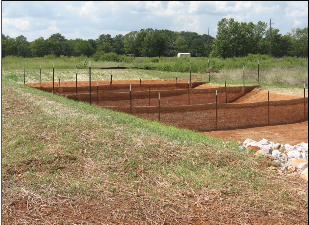
Figure SBN-3: Example of Porous Baffle Made of Coir Erosion Blanket as Viewed from the Inlet
