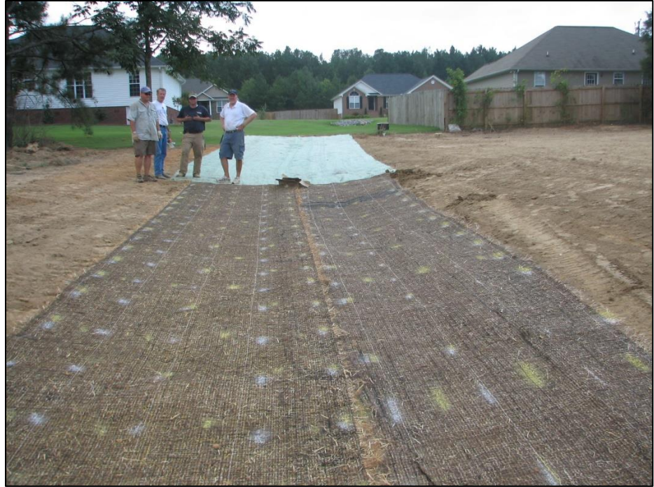
Figure ECB-4 TRM with Pre-Marked Stapling Pattern.
