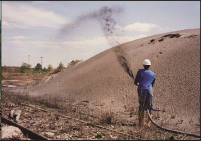
Application of Posi-Shell® via Extension Hose
