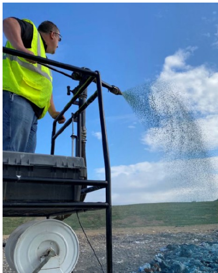
Application of VERDac Pellets via Deck -Mounted Discharge Wand
