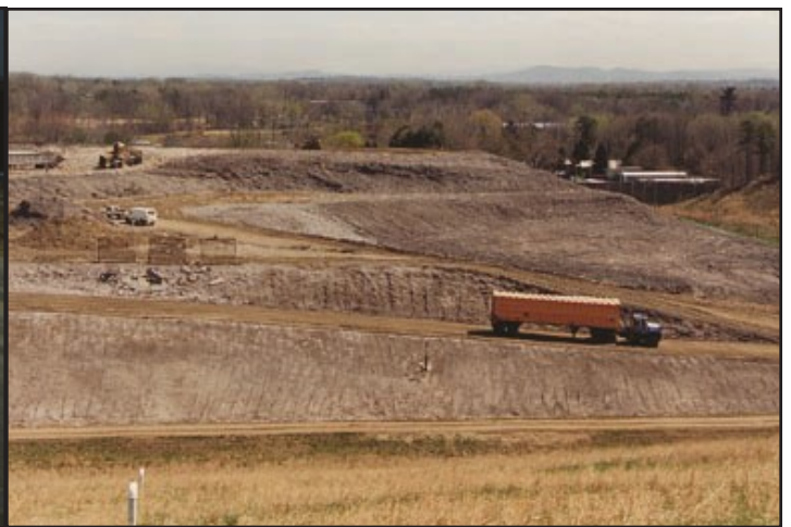
Finished Appearance of Posi-Shell® Intermediate Cover, Daily Cover, and Erosion Control at a Major Municipal Landfill
