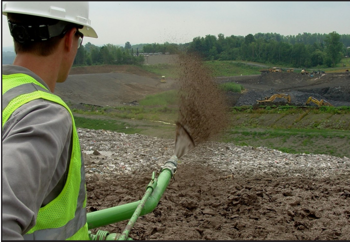
Application of Posi-Shell® via Deck-Mounted Discharge Wand
