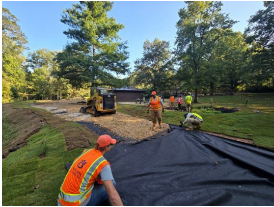
Figure 165- Crews working on implementation of LID in the park
