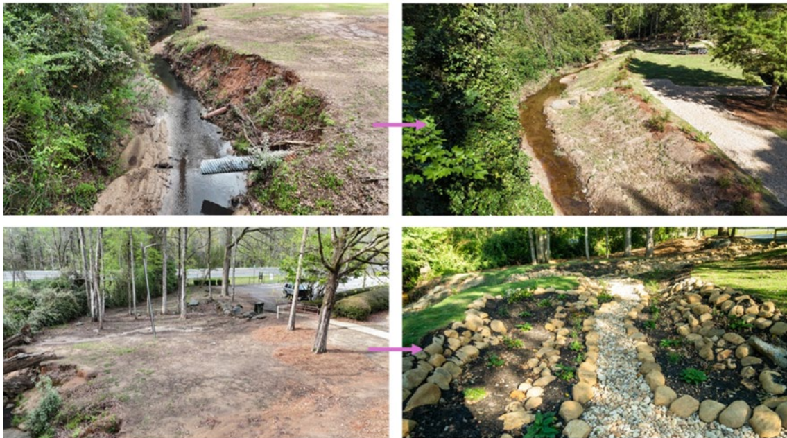
Figure 167- Before and After Pictures of Hickory Dickory Park with stabilization of slopes and flood plain creation as well as implementation of a bioretention area
