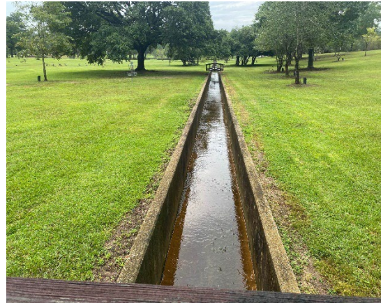
Figure 149 - Picture of concrete drainage structures that will be daylighted and a bioretention swale with sinuosity will be constructed in its place
