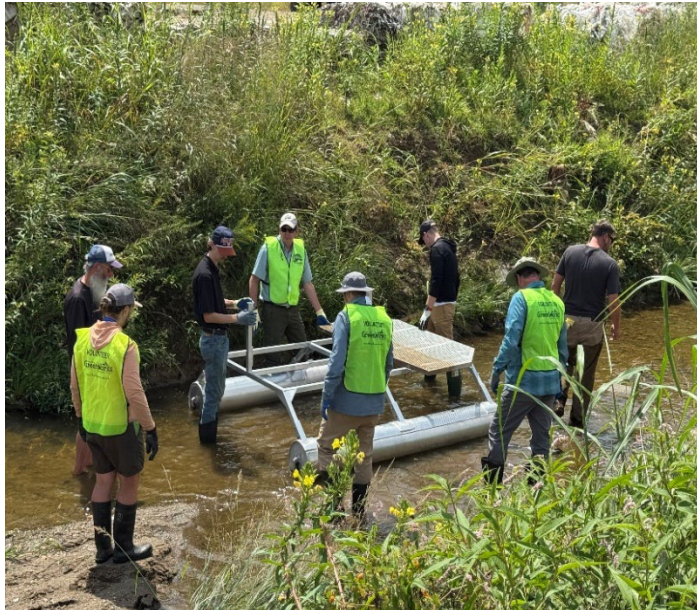
Figure 102- NPS Unit staff installing a litter trap in Nasty Branch
