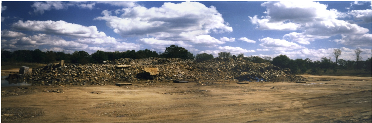
Foundry brick staged for removal
