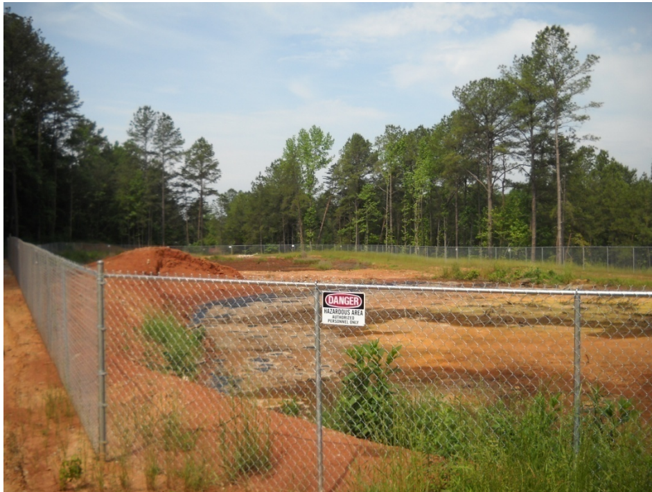
Completed slurry containment wall and enclosure
