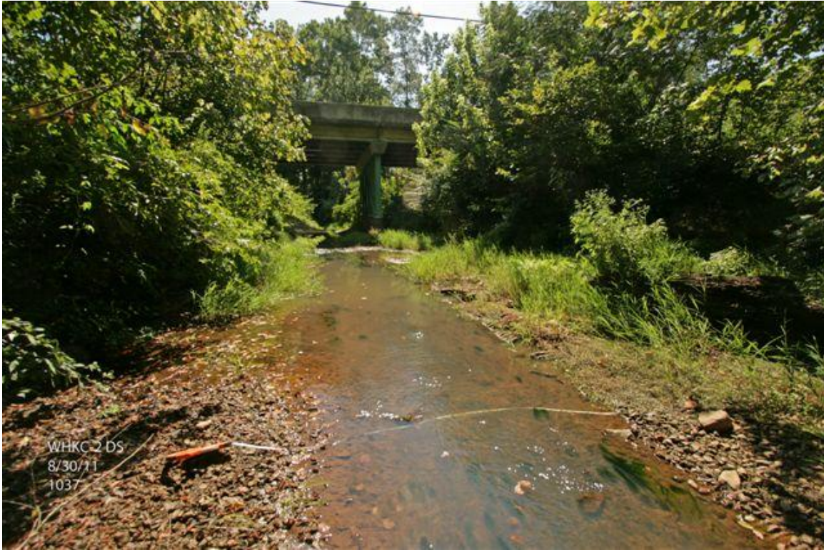
Figure 7: WHKC-2 Looking Downstream
