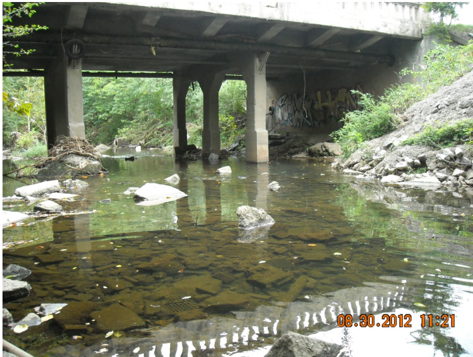
Photo 7-4 VLGJ-2 Looking Downstream
